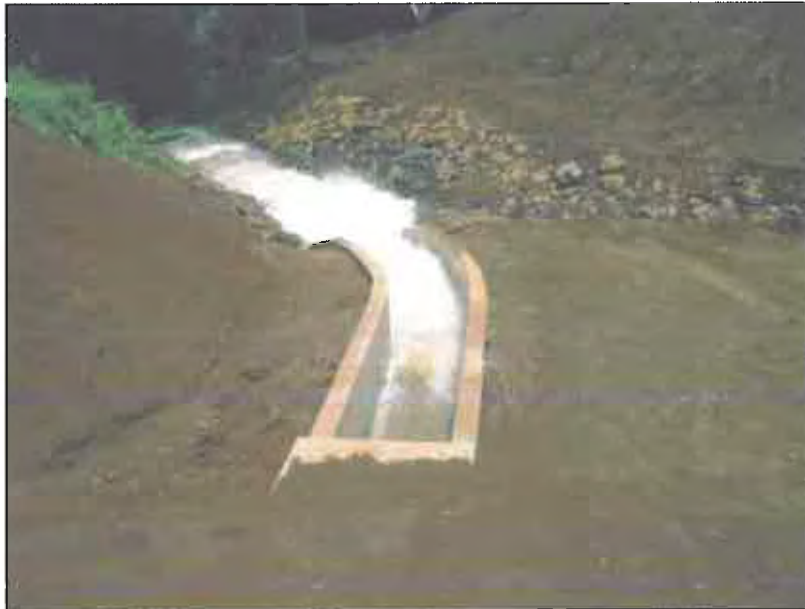
Spillway of O'Romis Power Station
