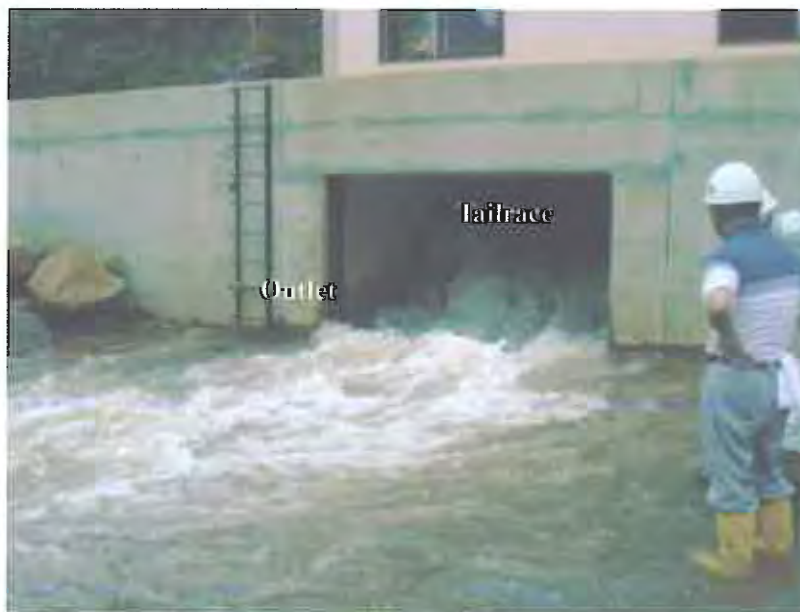
Tailrace of O'Moleng Power Station
