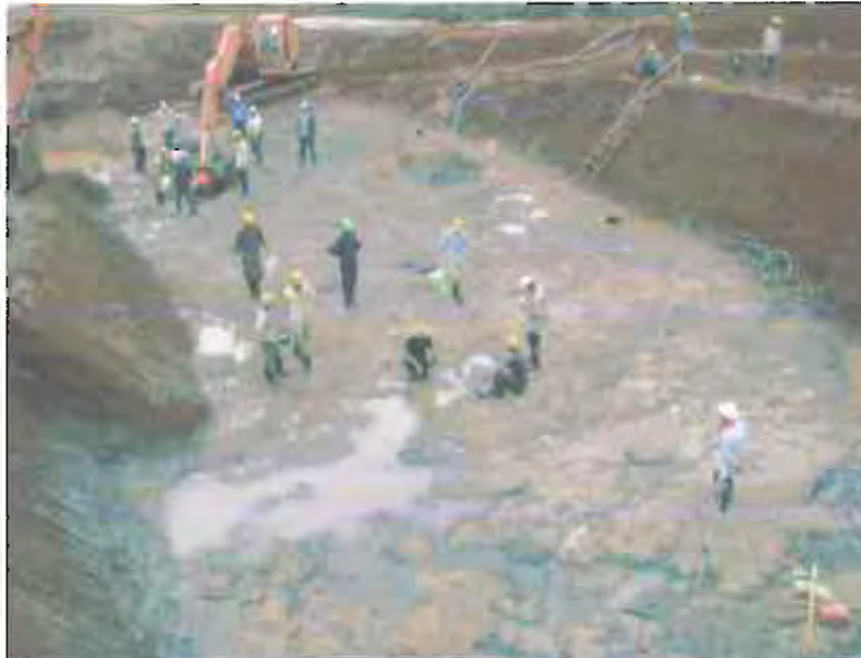
Example photo of intake weir basement (O’Moleng site)
