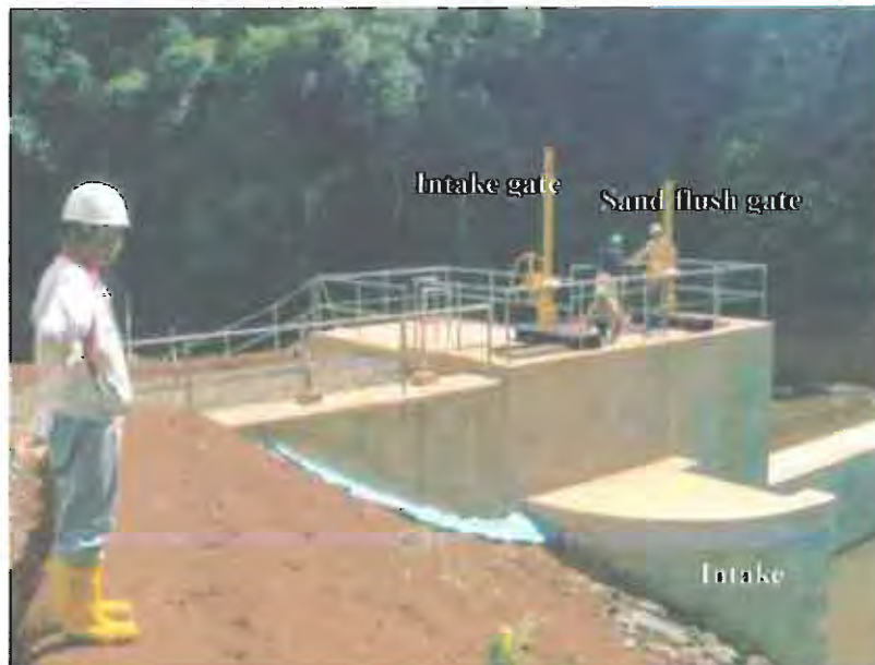
Intake of O'Moleng Power Station
