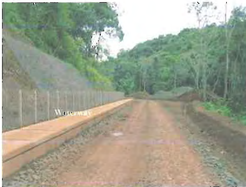
Waterway of O'Romis Power Station
