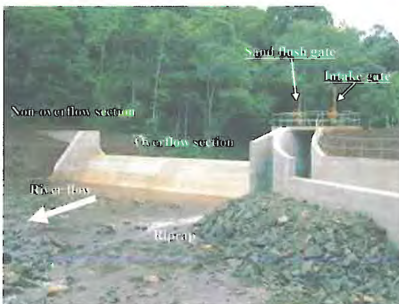
Intake Weir of O'Romis Power Station
