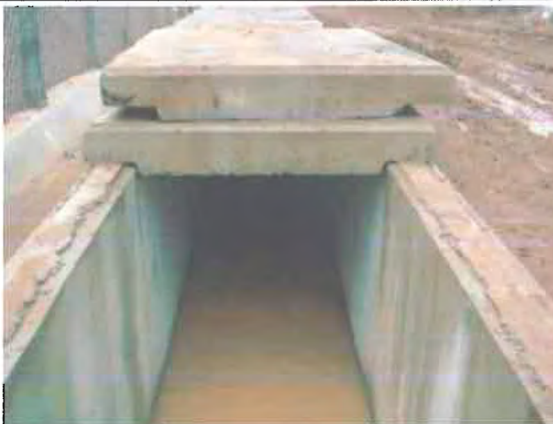
Inside of waterway of O'Romis Power Station
