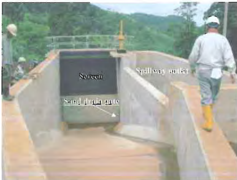
Head tank of O'Romis Power Station (No water)
