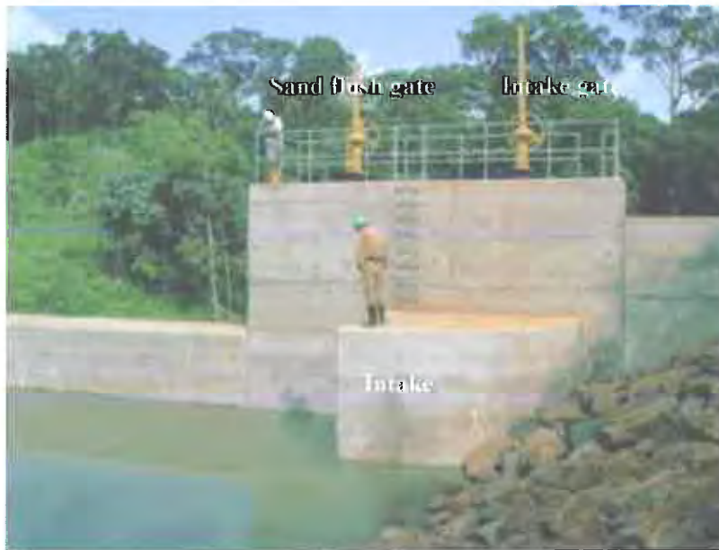
Intake of O'Moleng Power Station
