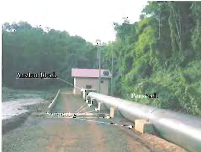
Penstock of O'Moleng Power Station (Exposed section)
