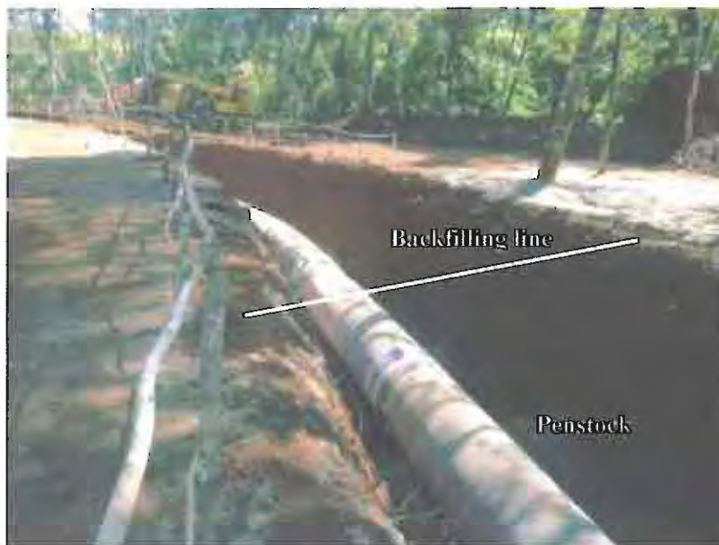
Penstock of O'Moleng Power Station (Buried section; under construction)
