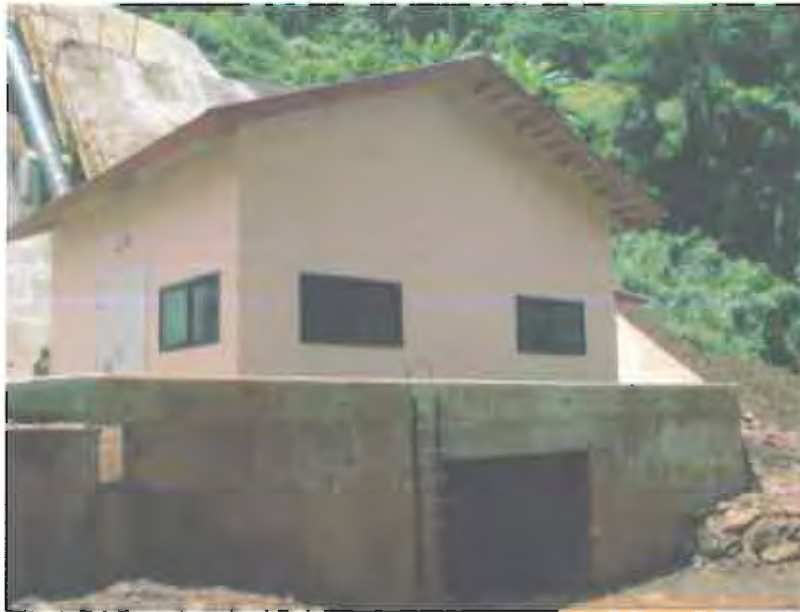
Powerhouse of O'Romis Power Station
