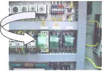
8) To insert a handle into Servomotor unit
