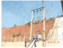
Step up Tr. at P.S (400V/22kV)
