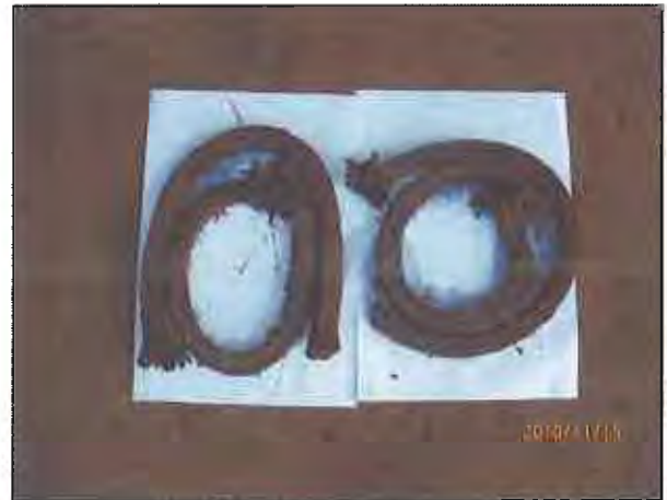
4. Used turbine ground packing
