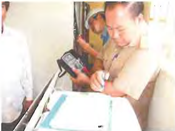
Measuring Insulation resistance of dummy load
