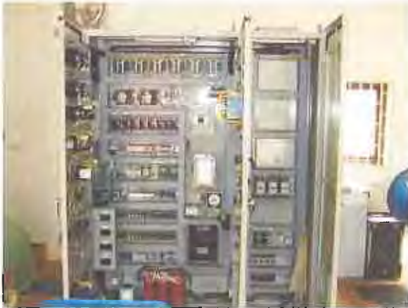
Inspection of Panel inside (Switches, meters and parts)
