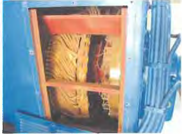
Inspection of inside Generator and cleaning
