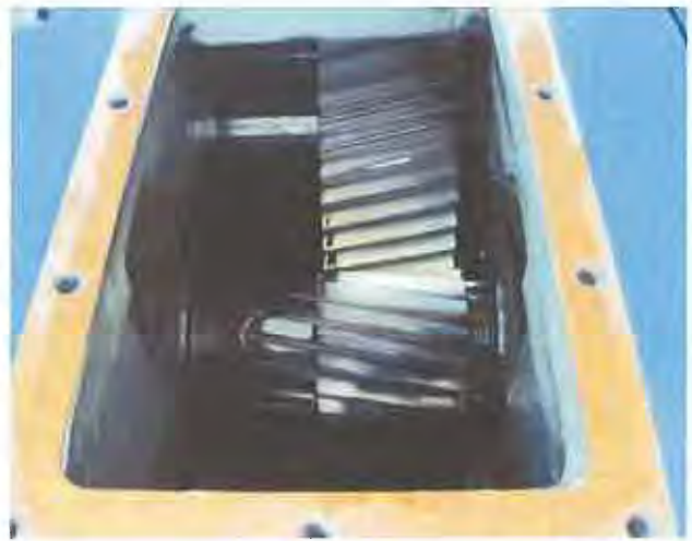
6. Inspection inside of speed gear
