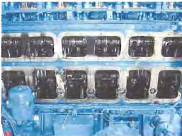
Inspection of inside Engine Room and Crank shaft
