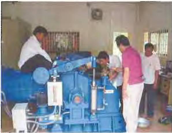
1. Disassembly work of turbine cover and
