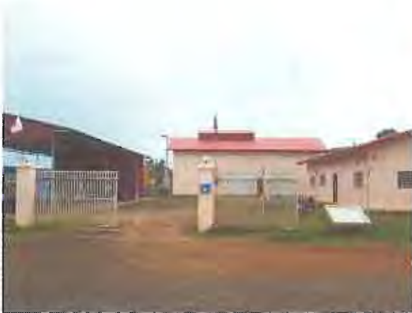
Administration and Diesel Generating Facility Buildings
