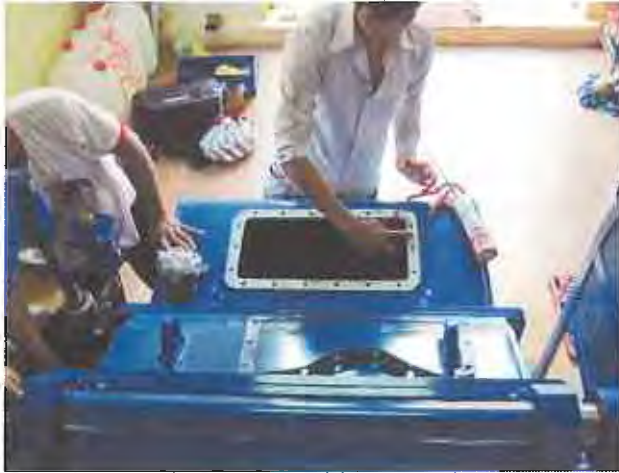
1. Disassembly work of turbine cover
