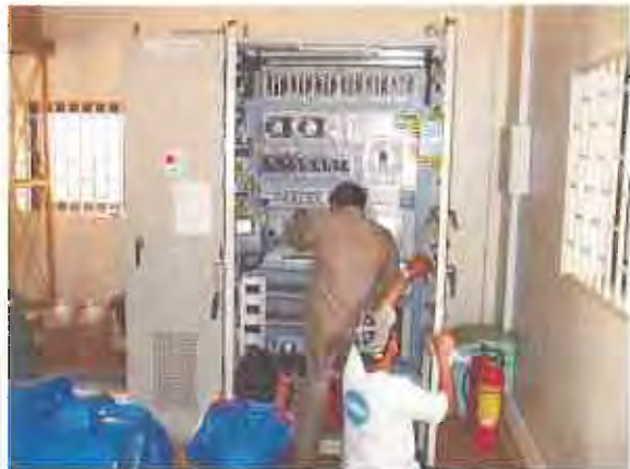
Inspection of cables connection and terminals at Control panels
