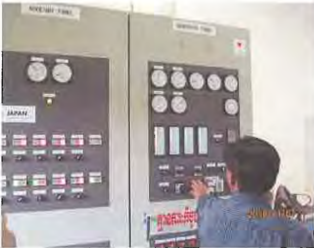
11. Trial operation after overhaul work
