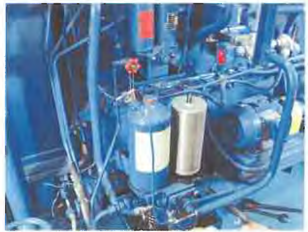
10. Cleaning of oil filters
