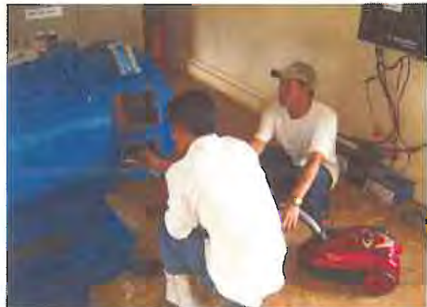
Inspection and cleaning of Generator inside
