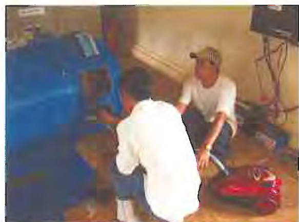
Inside inspection and cleaning of generator
