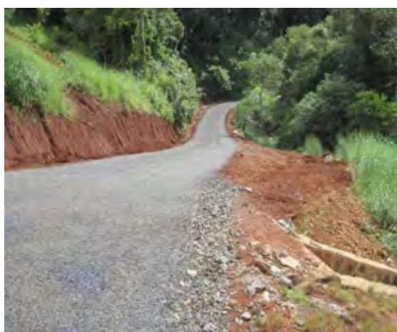
Access road to O’Romis (before)
