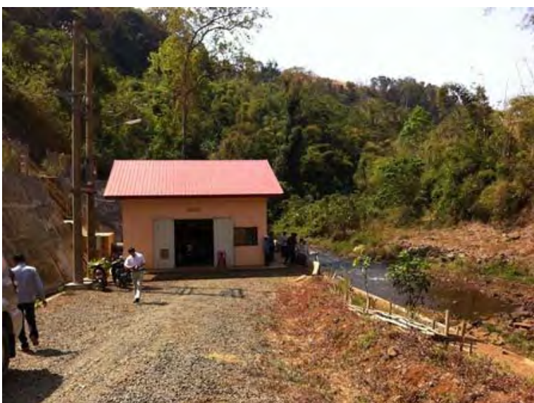
○ Status around O'Romis powerhouse
