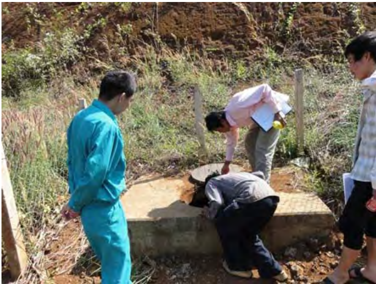
○ Patrol in progress (O'Moleng Power Station) Inspecting a manhole for the hydraulic pressure iron pipe
