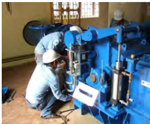
Servo-motor inspection at O'Romis P.S
