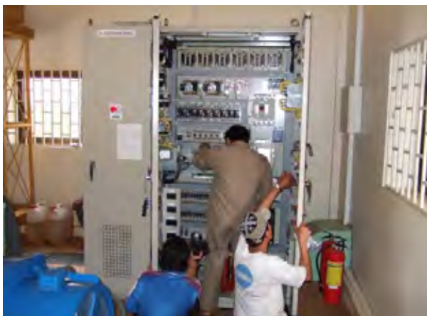
(Photo-left) Inspection and measurement of control panel
