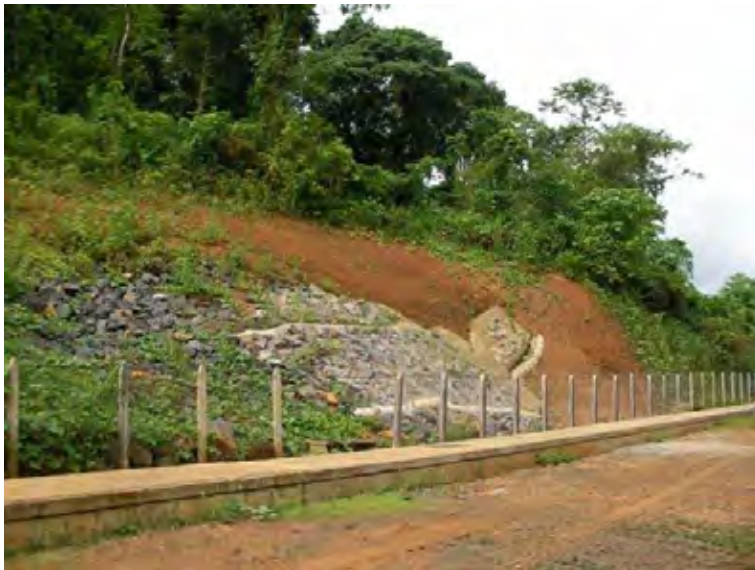
Repaired slope alongside the O'Romis Power Station access path
