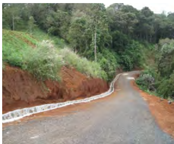
After repairing and pavement road
