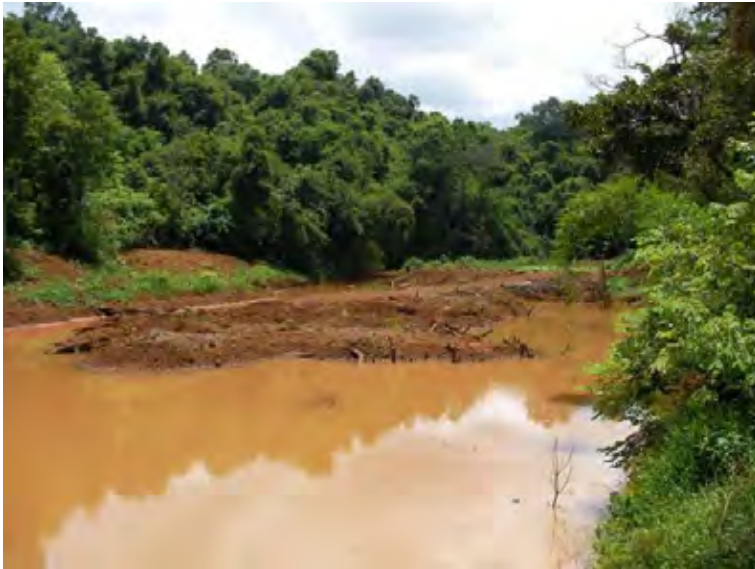
Temporary road left in the reservoir (Looking upstream from the diversion weir)
