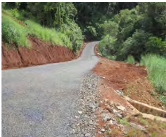
Access road from route 76 to O’Romis
