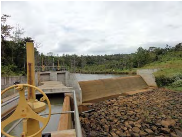
○ O'Moleng Power Station Present state of the diversion weir. There was no overflow from the weir. Hydropower when photograph taken: 100 kW.
