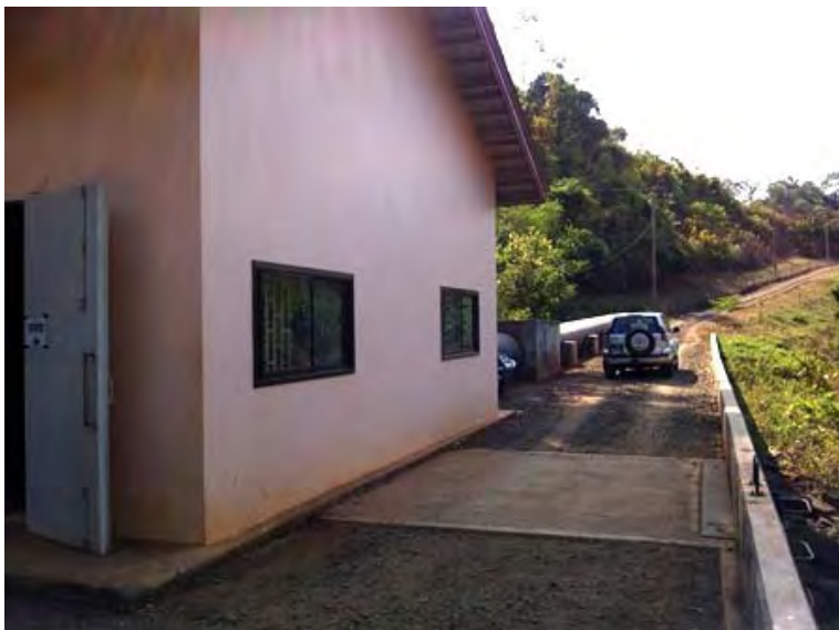
○ Status around O'Moleng powerhouse
