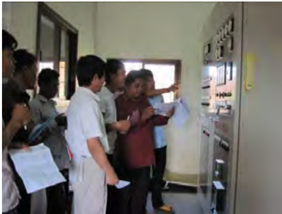
OJT at Control Panel
