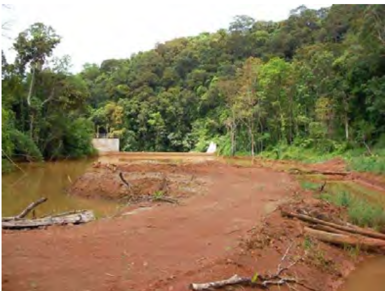
Same as above (Looking toward the diversion weir from the road)
