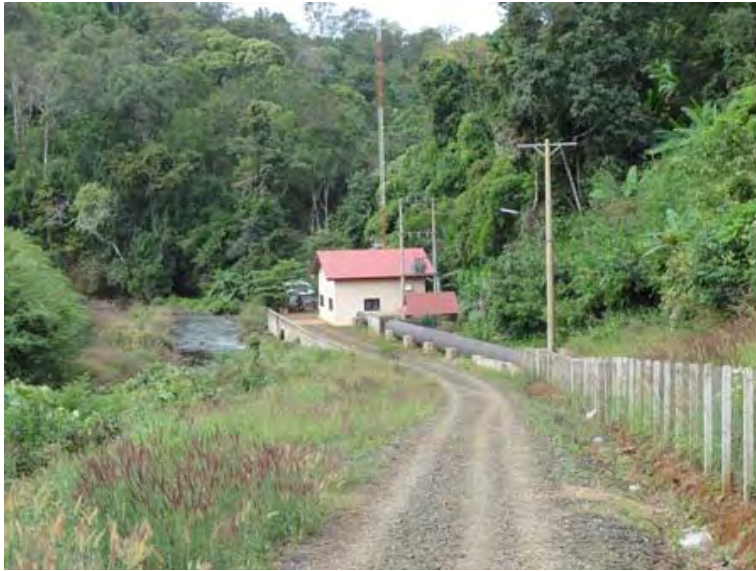
○ O'Moleng Power Station Present state of the power station
