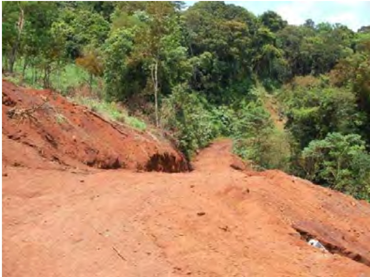
O’Romis Power Station entrance
