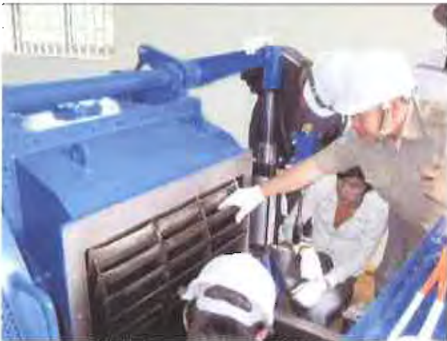
Inspection of turbine runner
