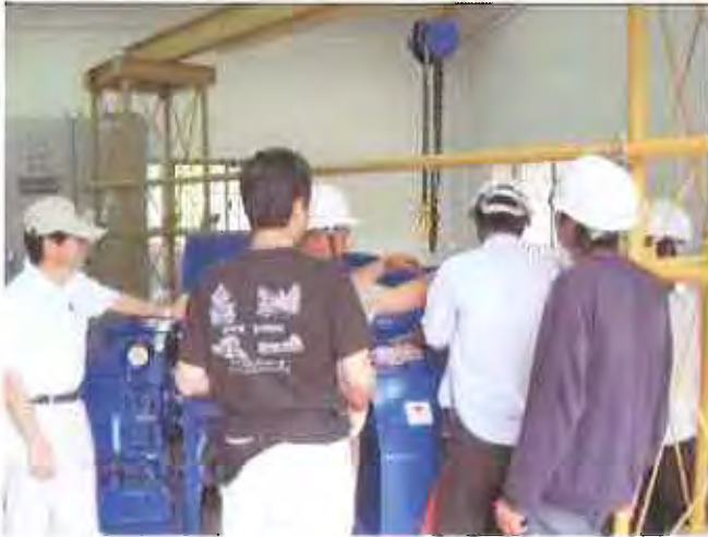
Disassembly of turbine cover
