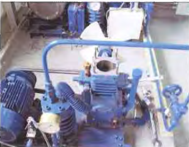
Disassembly inspection of air compressor
