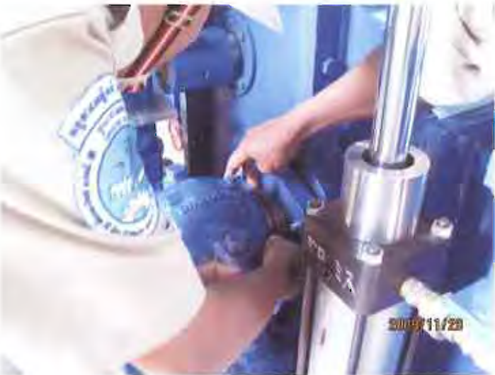
Disassembly of Ground Packing Cover for Turbine
