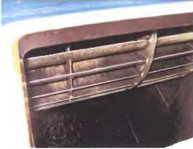
Turbine runner inside
