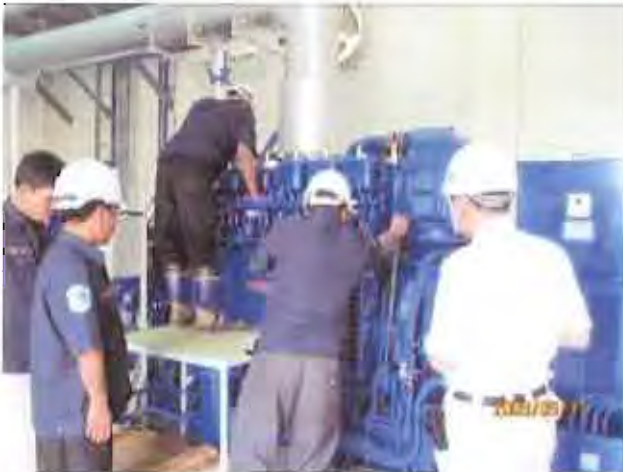
Timing adjustment by turning gear
