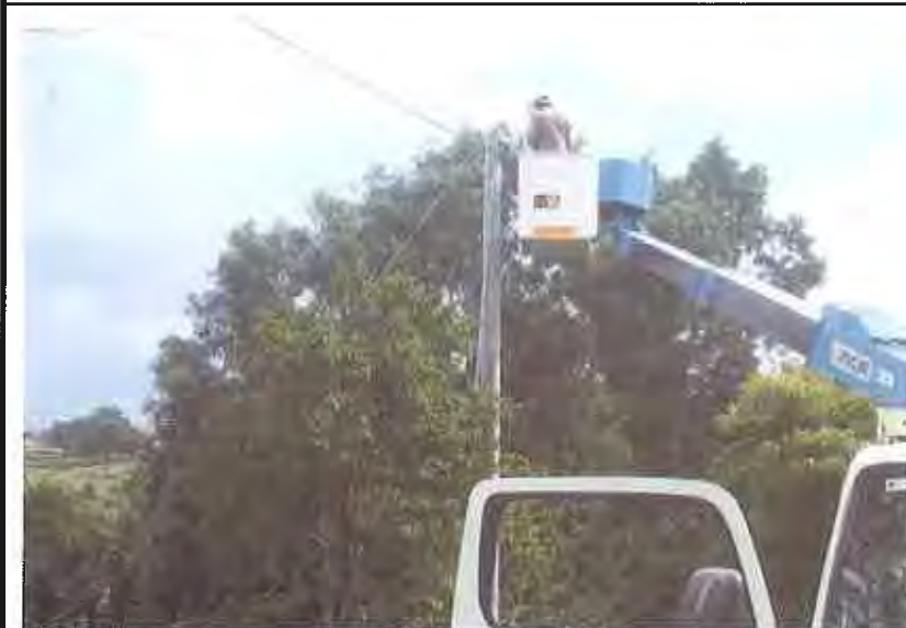
Training of low voltage distribution lines (400/230V) by Elevated work vehicle
