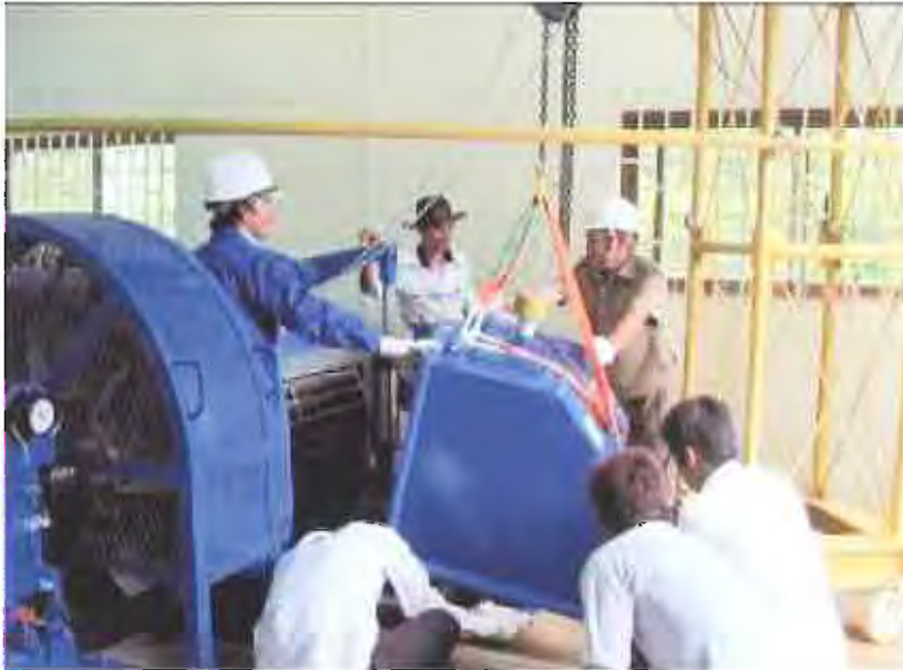
Periodic Inspection and OJT for Turbine Cover at O'Moleng Hydropower Station
