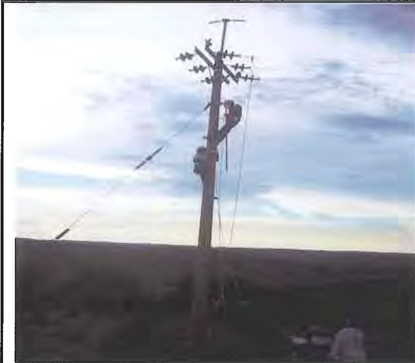
Repairing Work of Insulator on Concrete Pole
