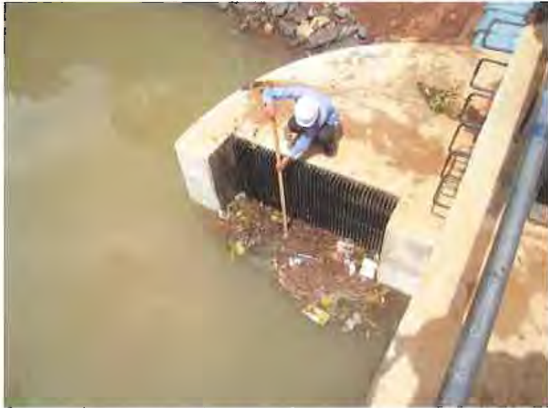
Cleaning Work at Intake, O'Romis Hydropower Station
