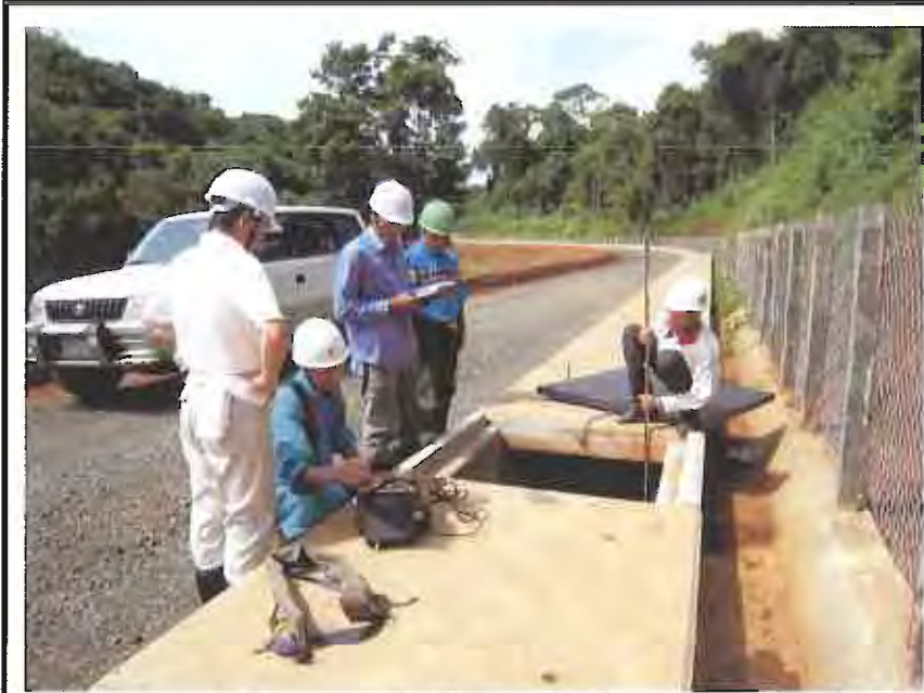
Measuring of Water flow at waterway, O'Romis Hydropower Station
