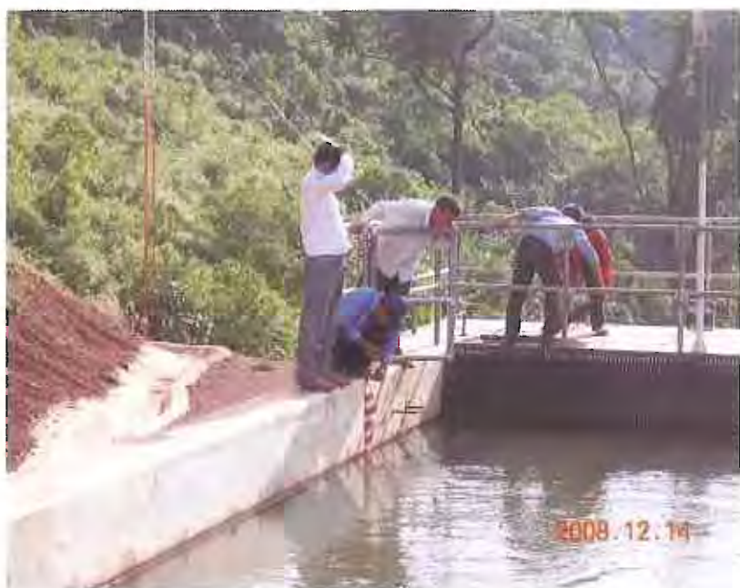
Measuring of water level at Head tank, O'Romis Hydropower Station
