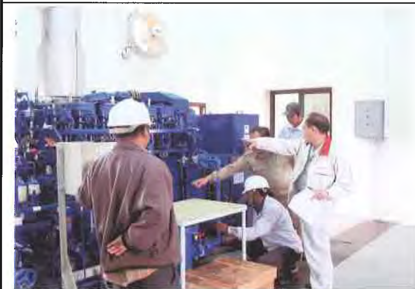
OJT for Weekly Inspection by Japanese Supervisor
