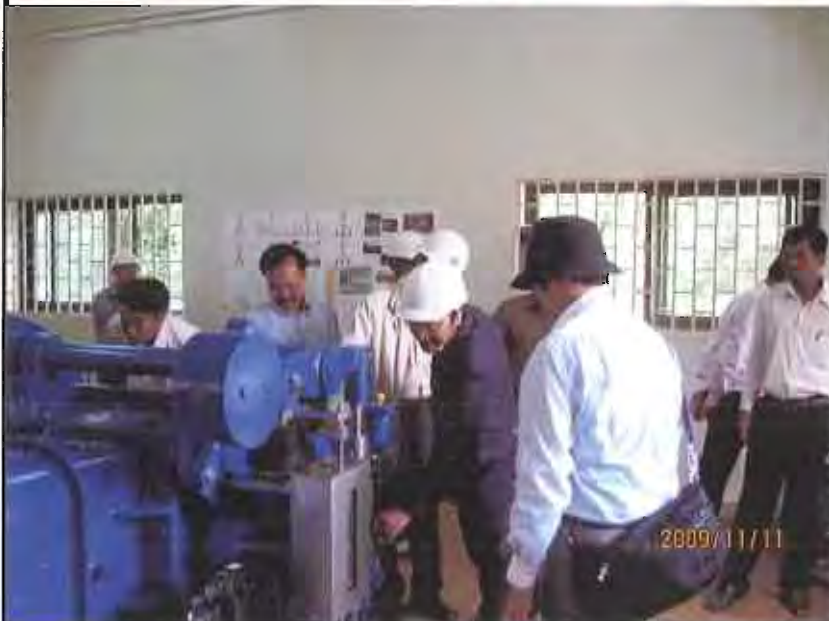
Defect Liability Test at O'Romis Hydropower Station by MIME/DIME and Contractor
