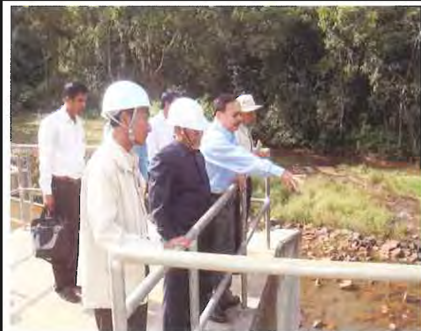
Defect Liability Test at O'Romis Hydropower Dam site by MIME/DIME and Contractor
