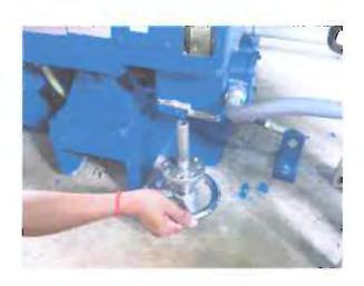
9) To confirm to do like this for 2 times. To charging Motor Spring by handle 52-2 (Indication "Red") To operate 52-2:0FF (Indication "Green) To charging Motor Spring by handle 52-2 (Indication "Green")
