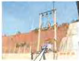
Step up Tr. at P.S (400V/22kV)
