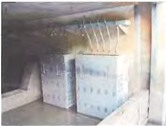
Assembly of Dummy load after cleaning
