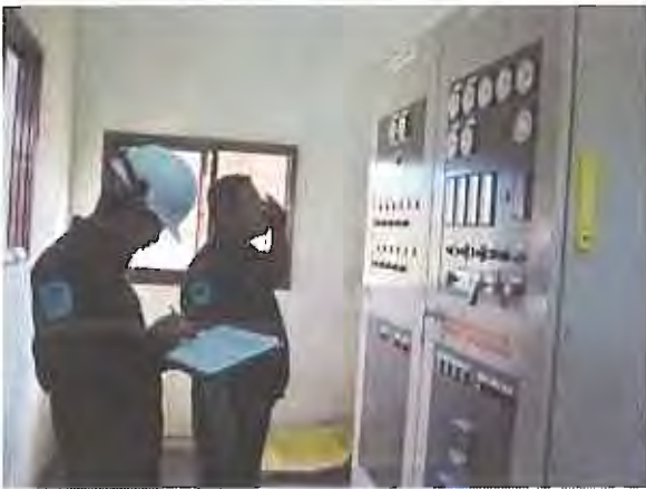
Trial Operation after Inspection
