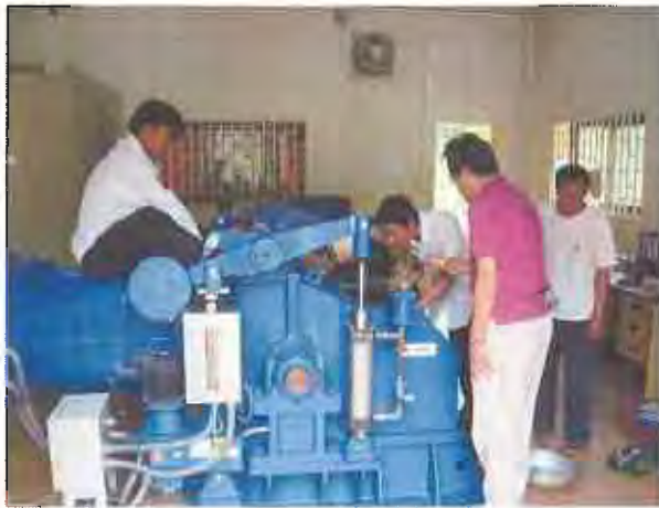
1. Disassembly work of turbine cover and
