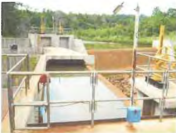
Drought condition at O'Moleng Hydropower station
