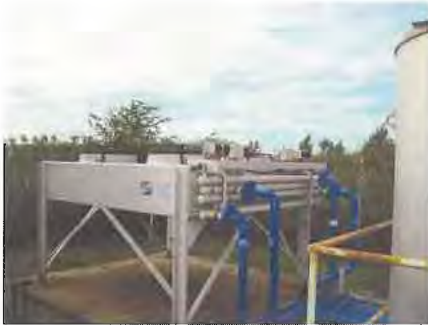
9. Inspection of cooler unit
