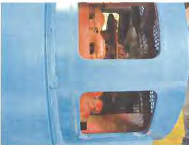
5. Cleaning of generator inside
