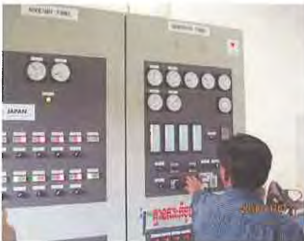
11. Trial operation after overhaul work
