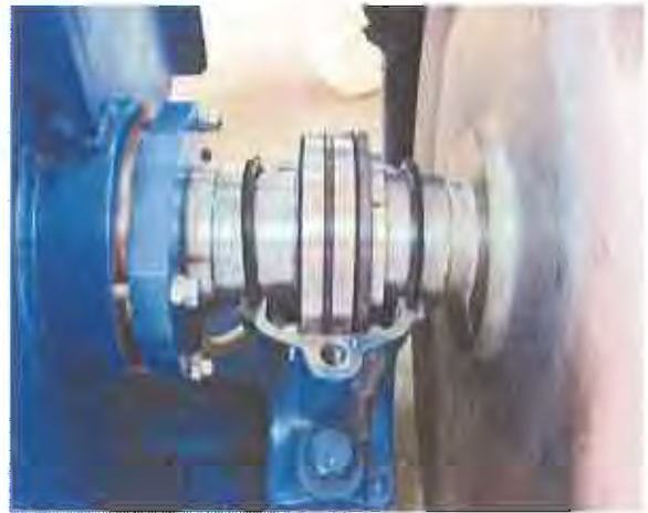
2. Cleaning of turbine bearings
