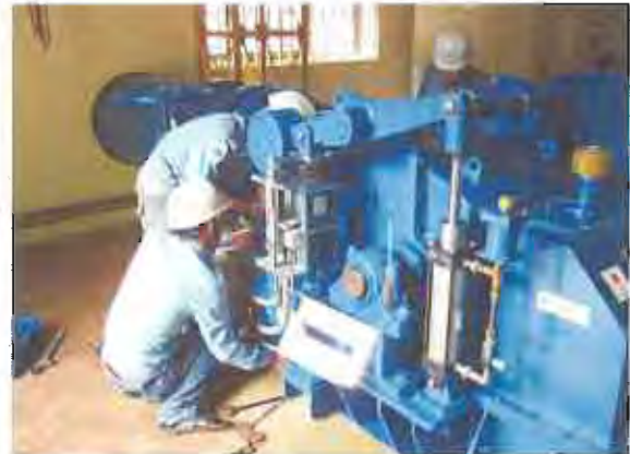
Adjustment of Servo-motor stroke for Guide-vane
