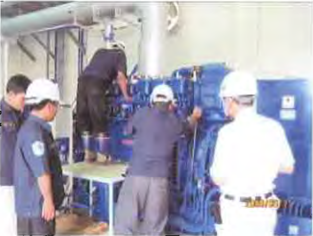
Timing adjustment by turning gear
