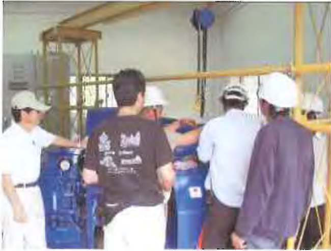
Disassembly of turbine cover
