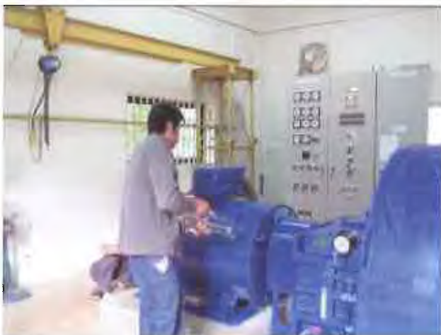
Grease up into generator bearings
