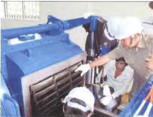
Inspection of turbine runner
