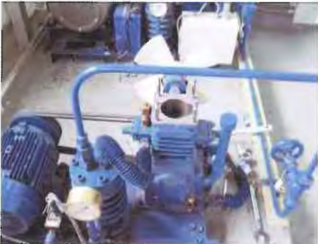
Disassembly inspection of air compressor
