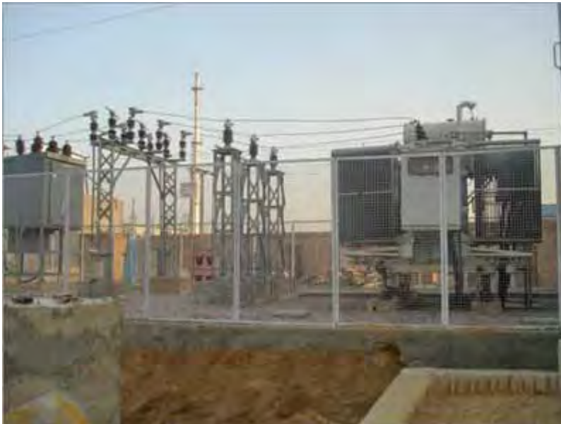
Figure 3: Typical Example of Substation Arrangement and Rehabilitation Work
