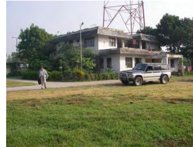
Existing Building where radio equipment room is located.
