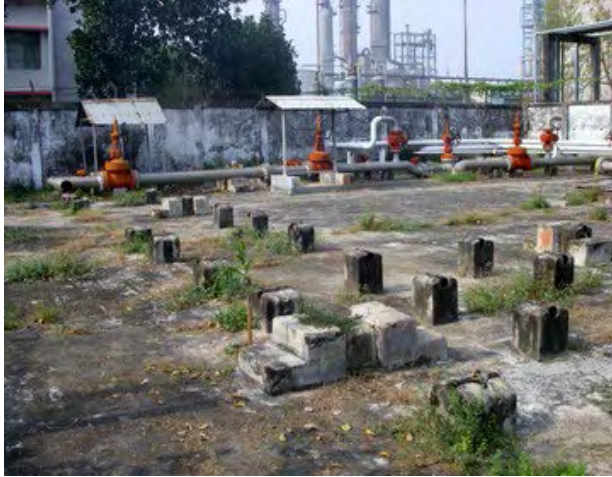
Old site where gas pipeline and instruments were removed.
