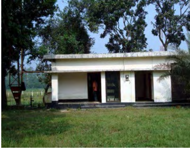
Existing Radio Building
