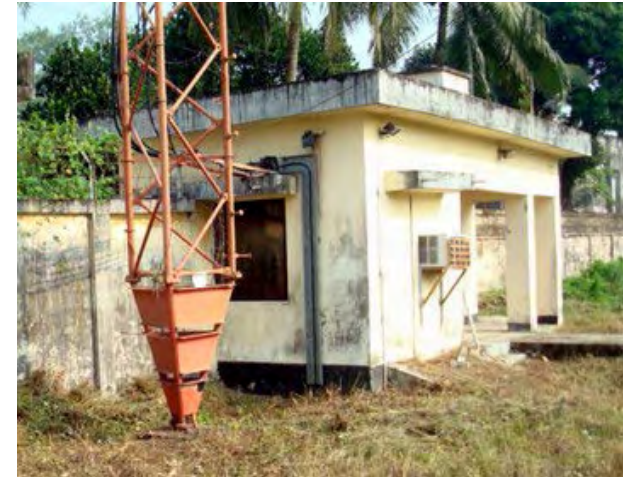
Existing Radio Building
