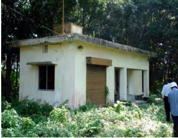
Existing Radio Building
