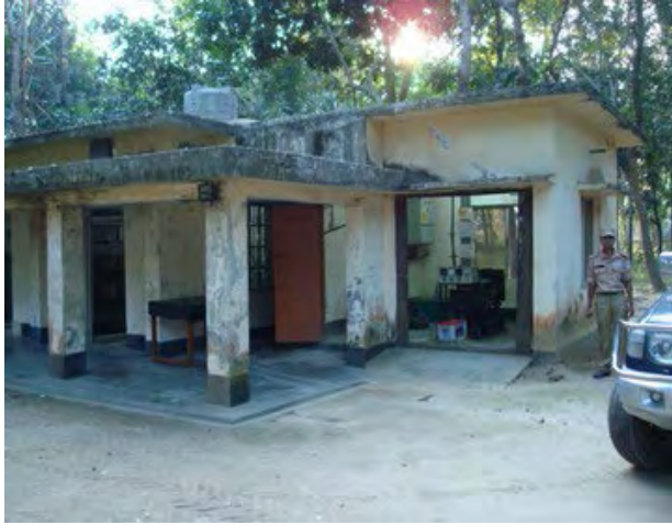
Existing Radio Building
