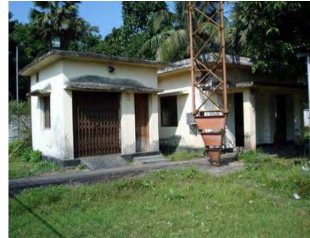
Existing Radio Building & Generator Room
