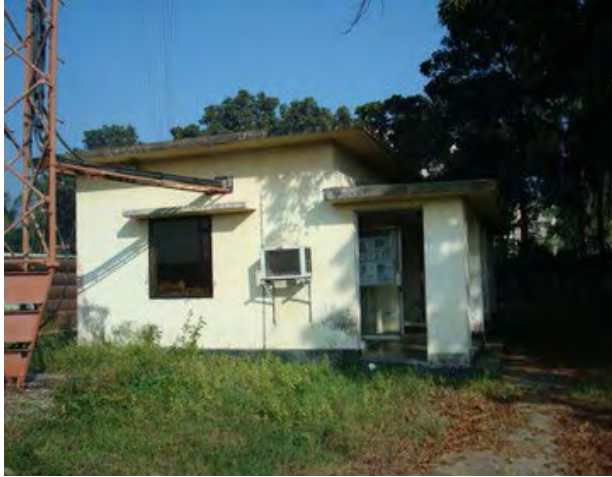
Existing Radio Building
