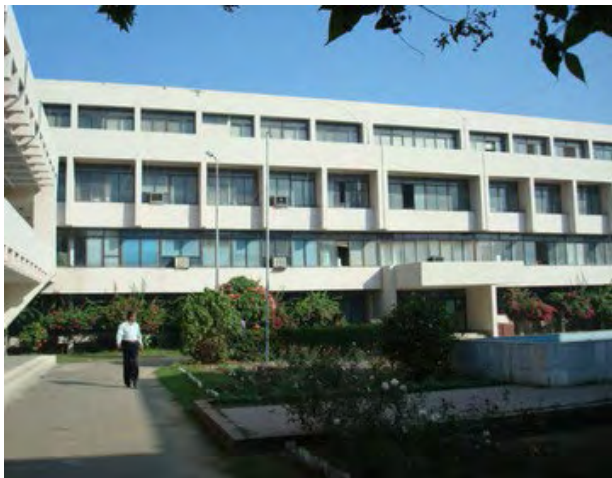
Comilla BGSL head office where new OCT shall be installed
