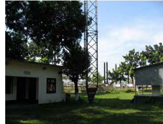
Existing Radio Building
