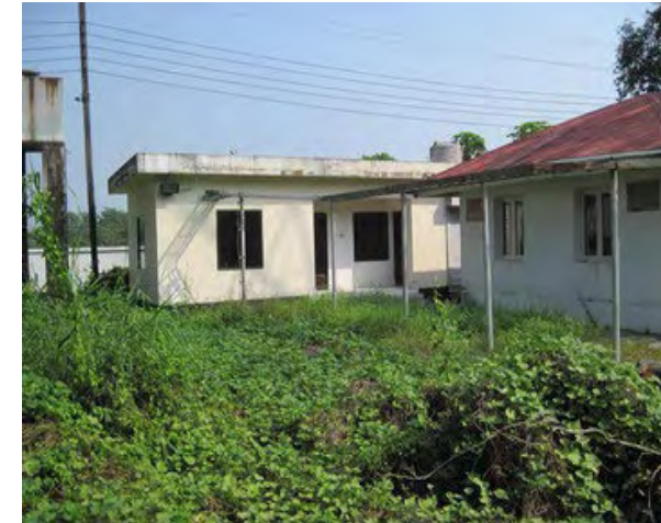
Existing Radio Building
