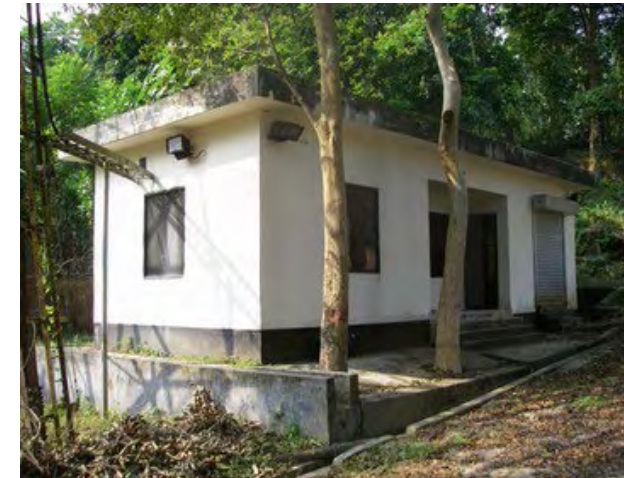
Existing Radio Building
