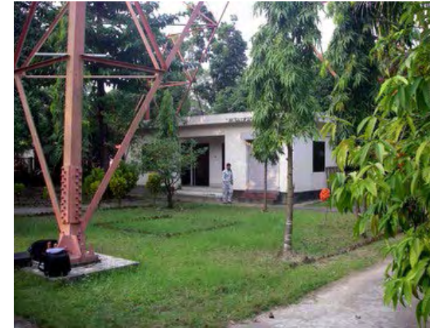
Existing Radio Building
