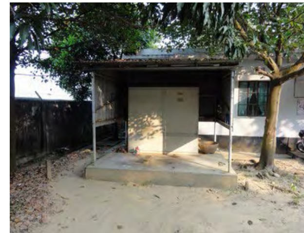
Existing RTU (cable link)
