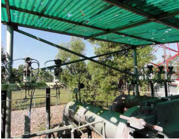
Site view with existing instruments
