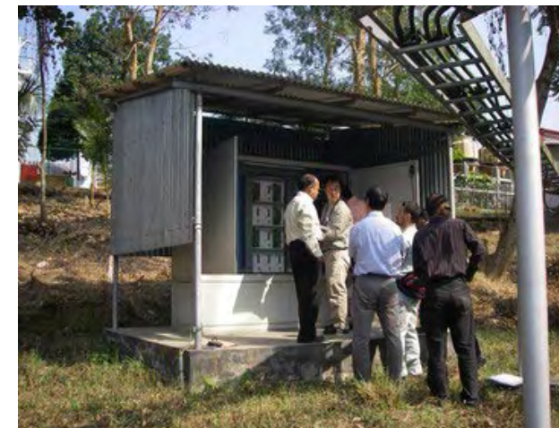
Existing RTU (cable link)
