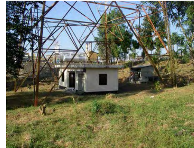
Existing Radio Building
