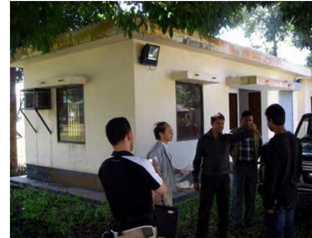
Existing Radio Building
