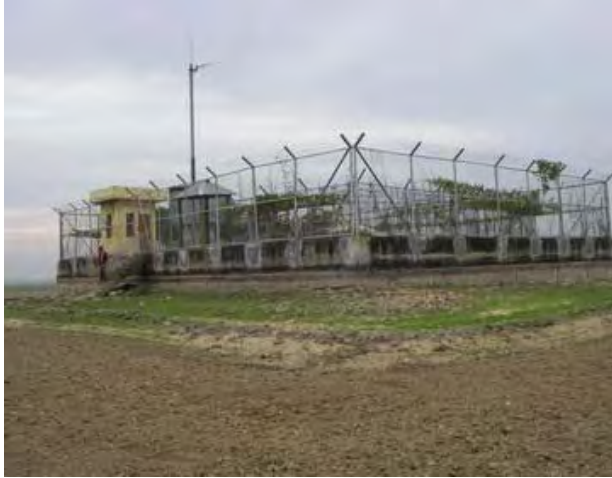
Whole view of site
