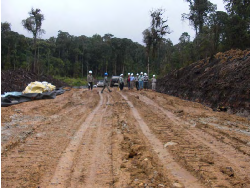
Access road between LMB2 cluster and LMB5 cluster (view toward north)
