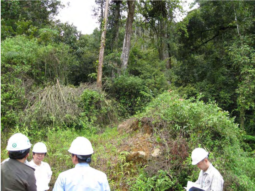
Access point of Unit 1 and Unit 2 power plant (View of power plant from access road)
