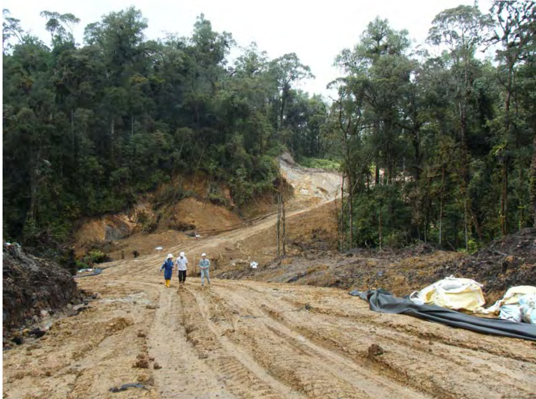
Access road between LMB2 cluster and LMB5 cluster (view toward south)
