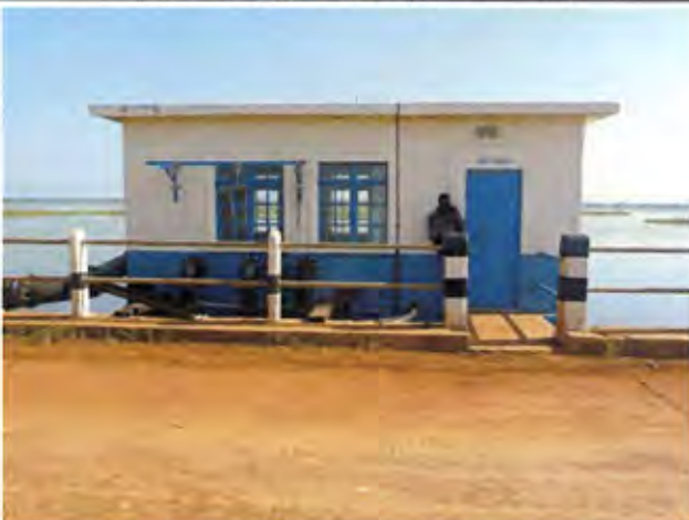
Intake facility for Soroti Municipality from Awoja River (Soroti District) [June 2009]
