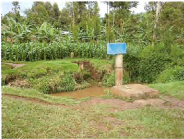
River gauging station (Sironko District) [June 2009]
