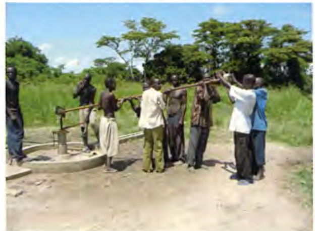
Repair works of handpump (Soroti District) [Jul. 2009]
