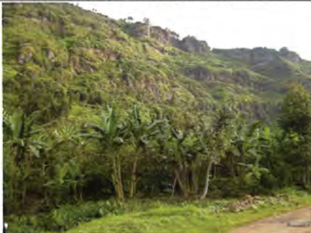
Sediment disaster site near Mbale (Mbale District) [June 2009]
