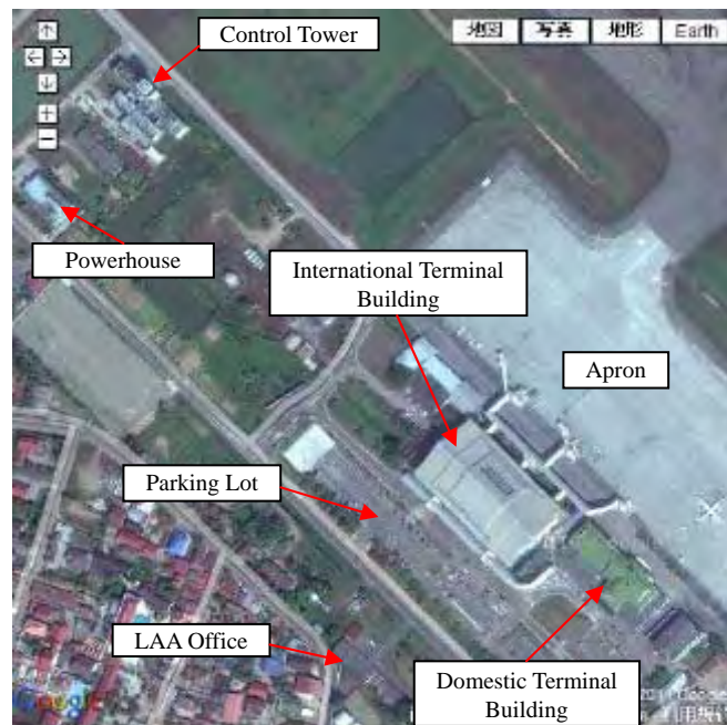
Fig. 1-2.2 Overall Photo of Wattay International Airport
