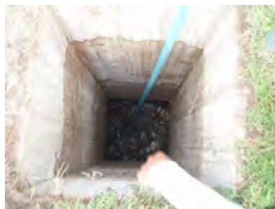
View from Manhole-1
