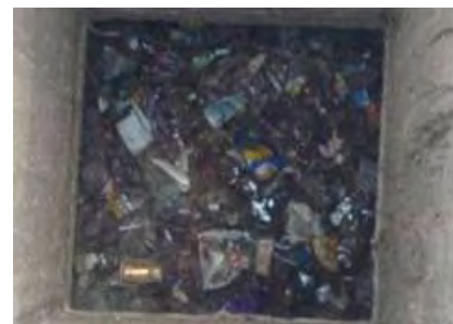
View from Manhole-2
