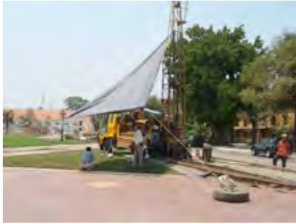
(At Boring Works)
