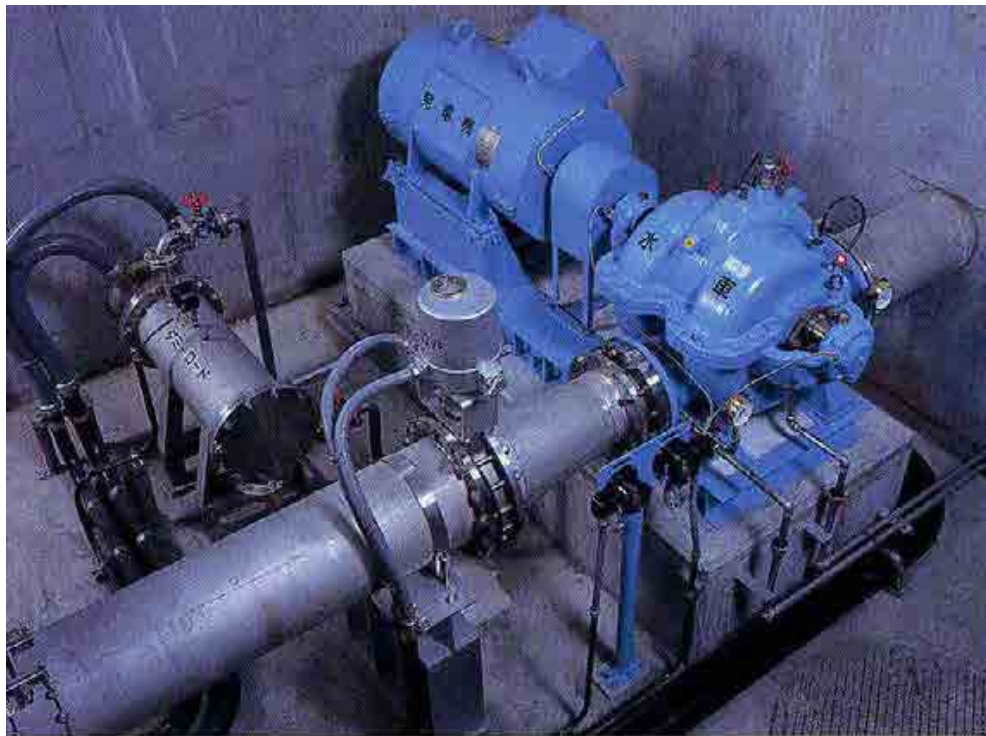
Figure 10-16 Reverse Pump Turbine(Double Suction, Single Stage, Volute Pump)
