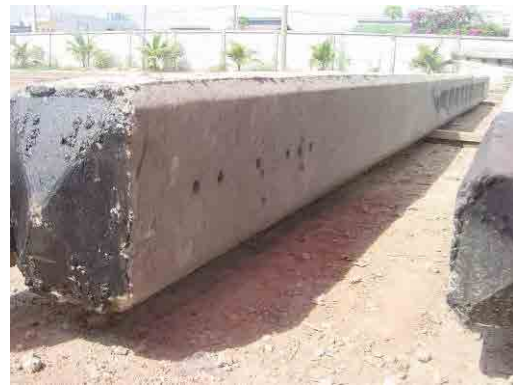
Figure 11-7 Reinforced Concrete Pole (Rectangular)
