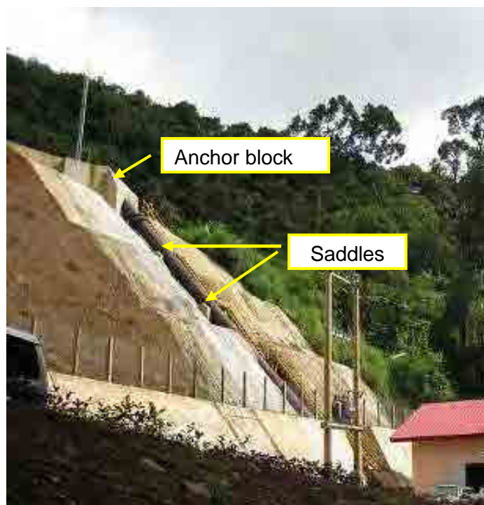
Figure 9-13 Example of Penstock
