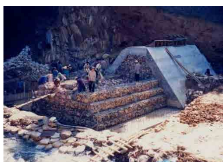
Figure 9-2 Concrete Reinforced Gabion Dam
