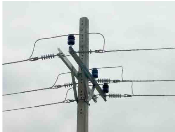
Figure 11-10 Insulators (Pin Insulators are Porcelain, Strain Insulators are Polymer.)
