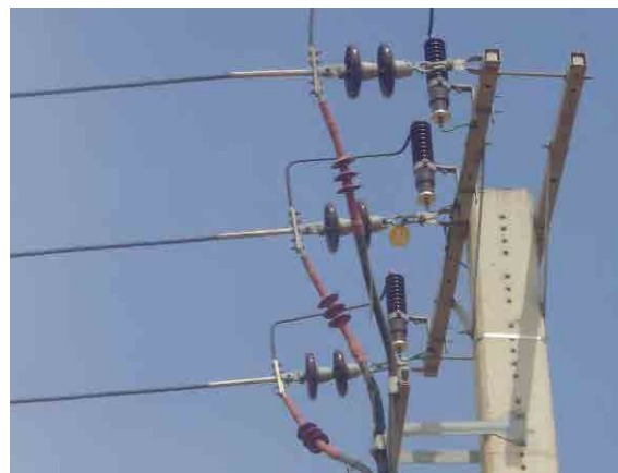
Figure 11-19 Arresters (for Cable Head Protection)
