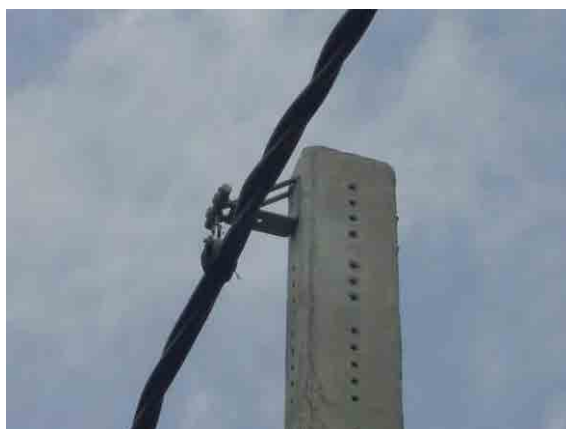
Figure 11-9 Cable Supported by Rack Hardware
