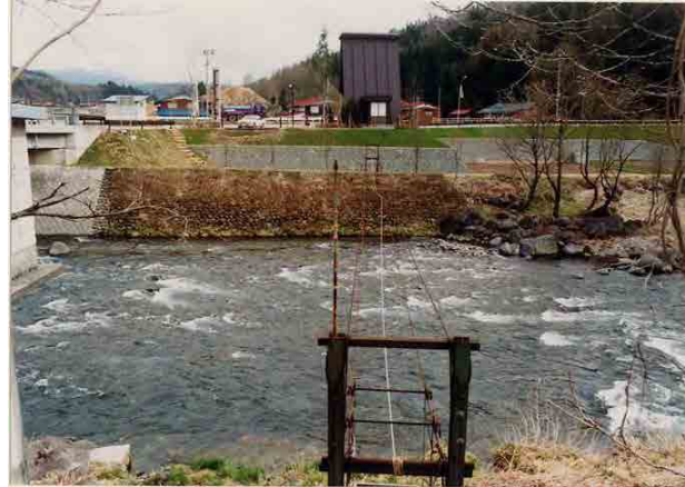
Figure 9-23 Flow Gauging Station
