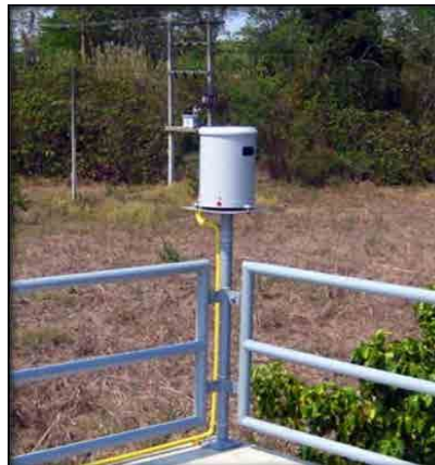
Figure 9-21 Example of Rain Gage Installation
