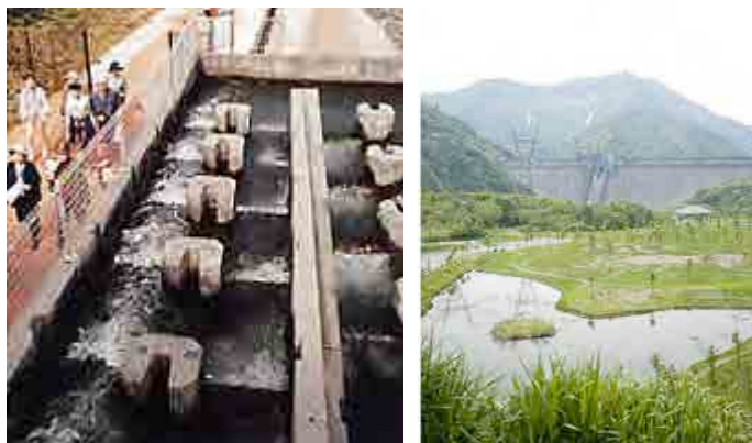
Figure 15-7 Example of Fish Pass and Biotope
