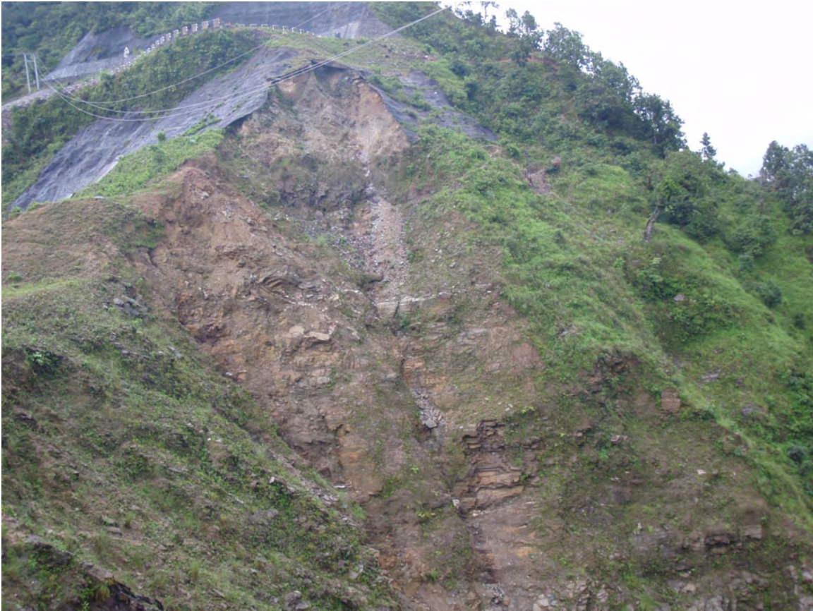
Photo.3 Full view of a failure at Sta.18+200 site. (from Sta.17+400)
