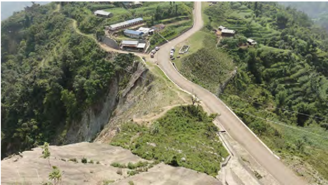
Photo.2 Full view at Sta.17+400. (from Sta.18+200)
