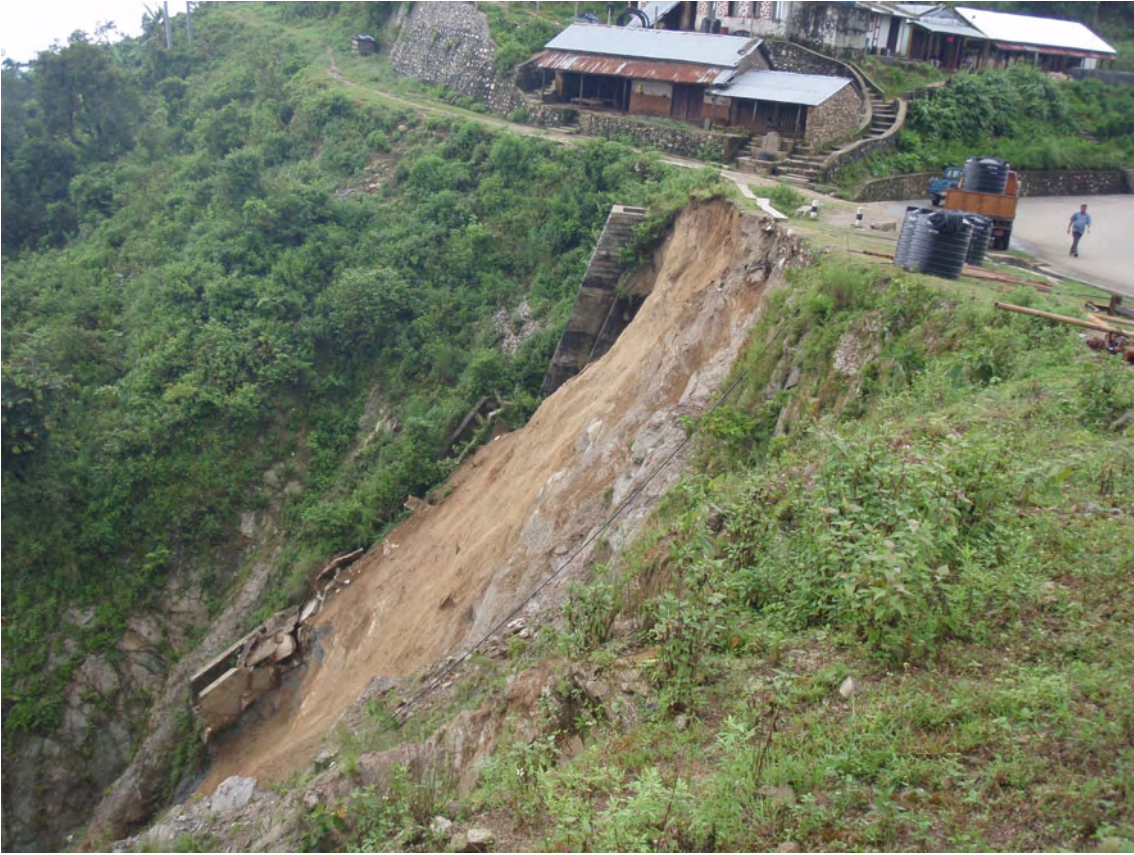
Photo.6 Surface failures at Sta.17+400.
