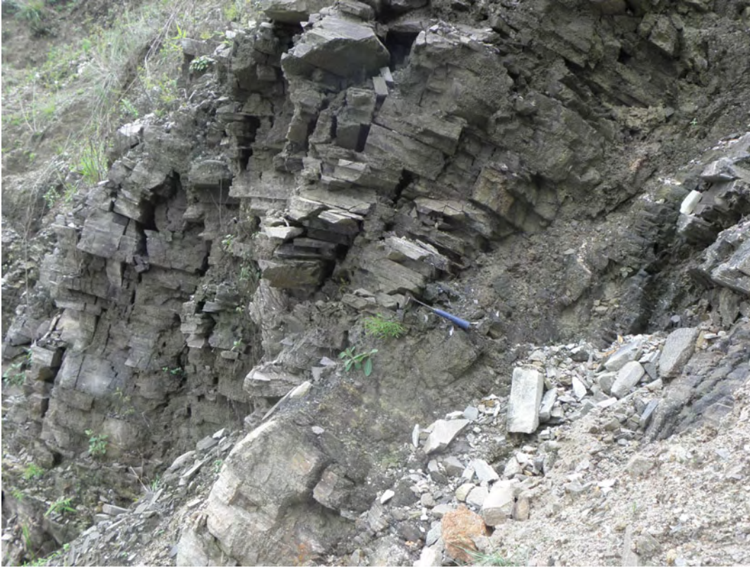
Photo.8 Unstable bedrock due to creep at Sta.18+200.
