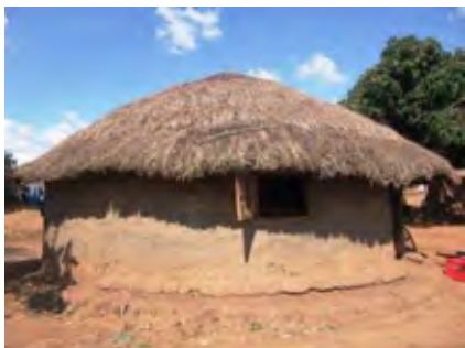
Temporary house, grass thatched roof with walls made of mud in Masindi
