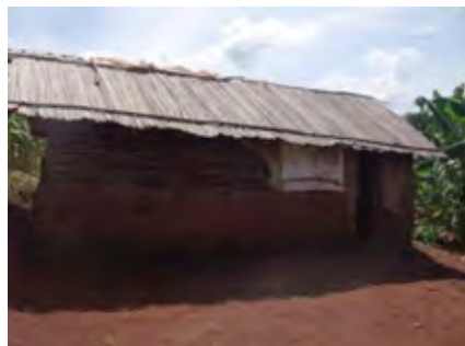
Temporary house, roofed with iron sheets with walls made of mud in Masindi
