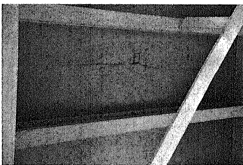
Figure 3.3.31 Krung Thep Crack (steel plate at the bottom surface of a deck)
