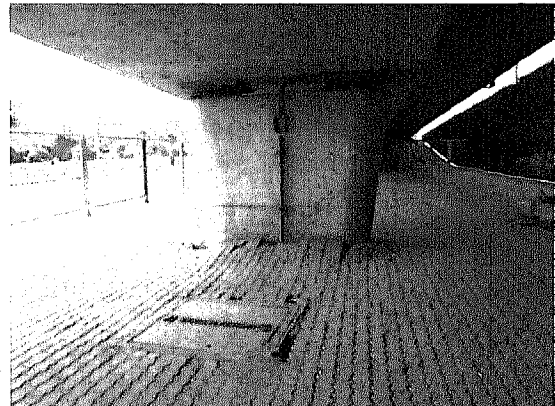
Figure 3.3.8: Ground settlement around Rama 5 (Thon Buri side)
