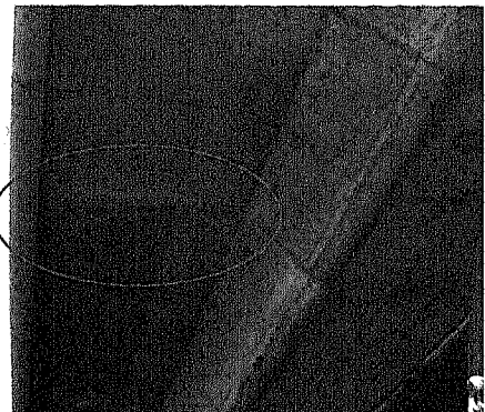
Figure 3.3.6: Cracks and free lime in Rama 5 (Bottom surface of projected deck)
