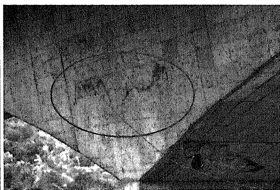
Figure 3.3.17: Cracks in the Phra Pokklao (Web of main girder)
