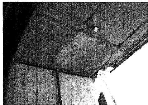
Figure 3.3.3: Free lime of Rama 4 (Lower Flange of girder)
