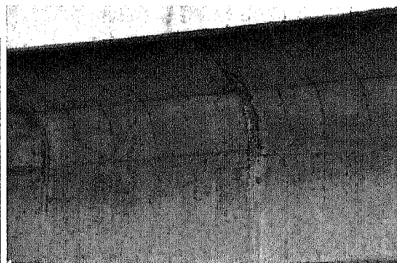
Figure 3.3.14: Phra Pinklao (Cracks and free lime on girder)
