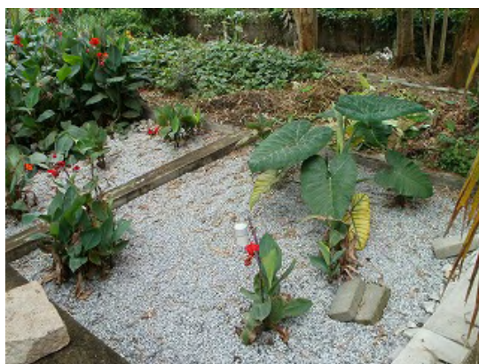
Biological aerated filter
