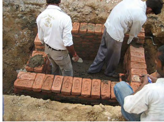
Collect Chamber Construction
