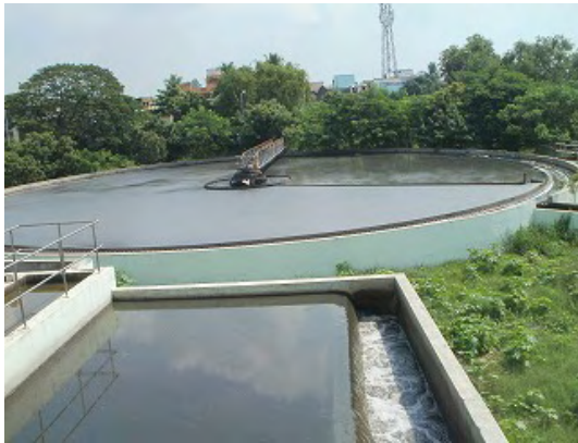
Primary sedimentation tank
