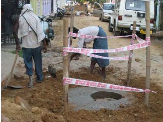
Collect Chamber Construction
