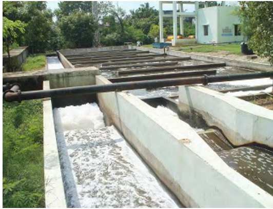
Chlorination chamber
