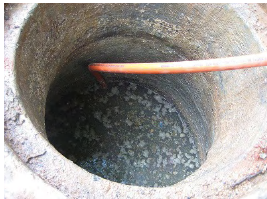
Situation of Cleaning
