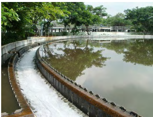
Final sedimentation tank
