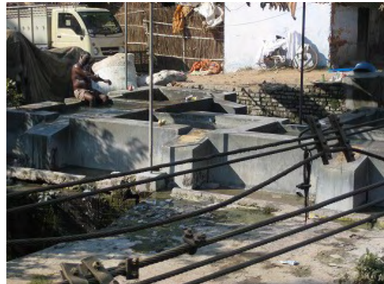
Drainage from a public wash place
