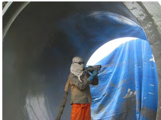
Lining of sewer pipe
