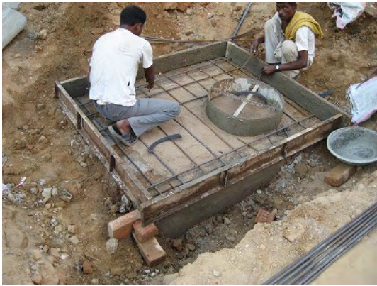
Collect Chamber Construction
