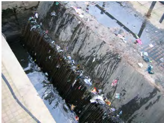
Solid waste reaching screen before grit channel
