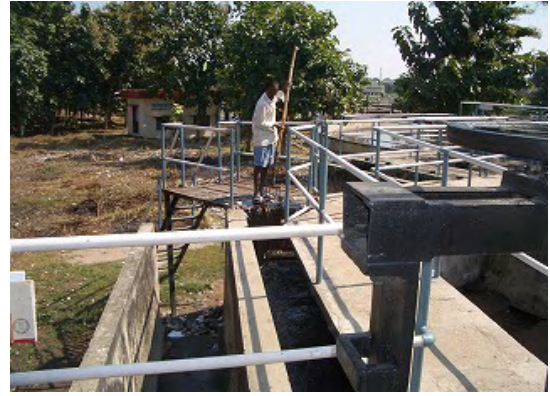
Fine screen operated manual
