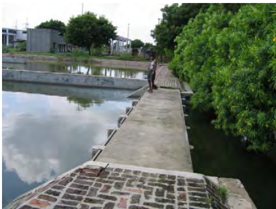
Outlet of polishing pond
