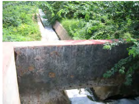
Final effluent channel
