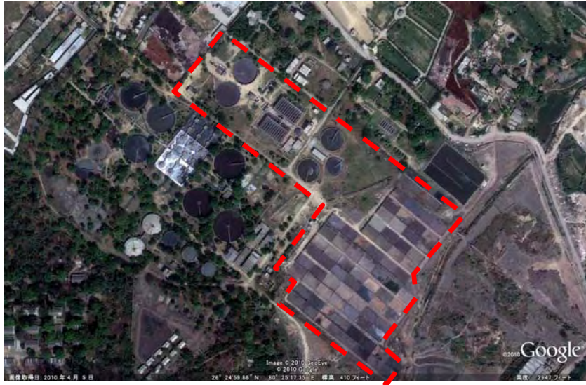
Figure 36 Location of 36 MLD STP in Kanpur
