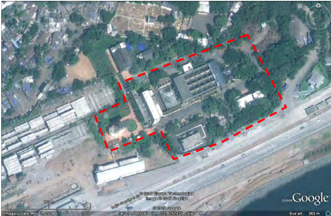
Figure 24 Location of Treatment Facilities at Bandra Outfalls
