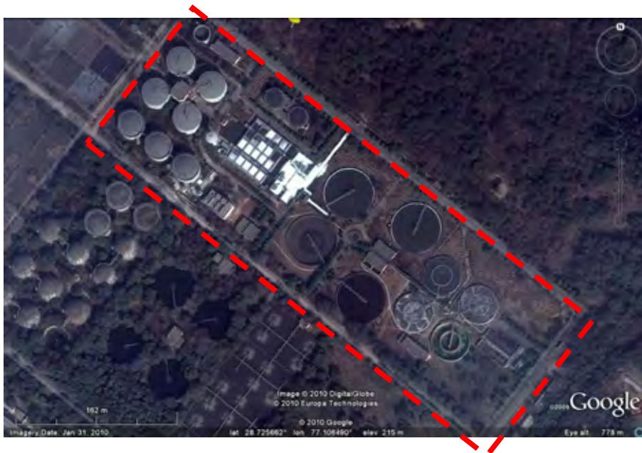
Figure 3 Location of Rithala STP (Phase II)
