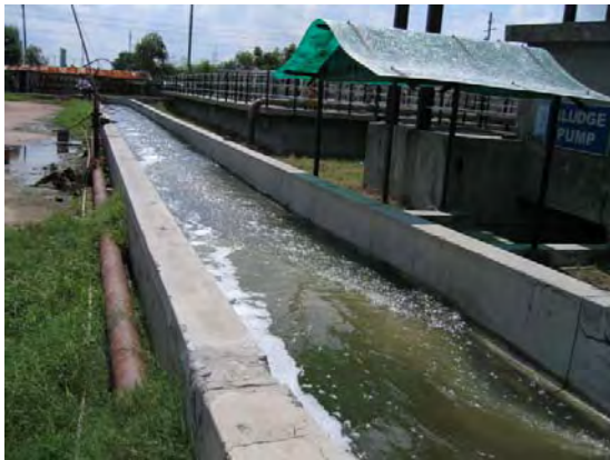
Effluent channel from UASB flowing to polishing pond
