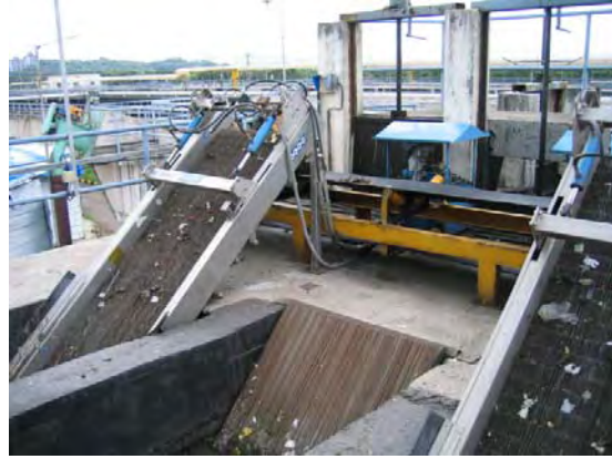
Fine screen operated mechanically
