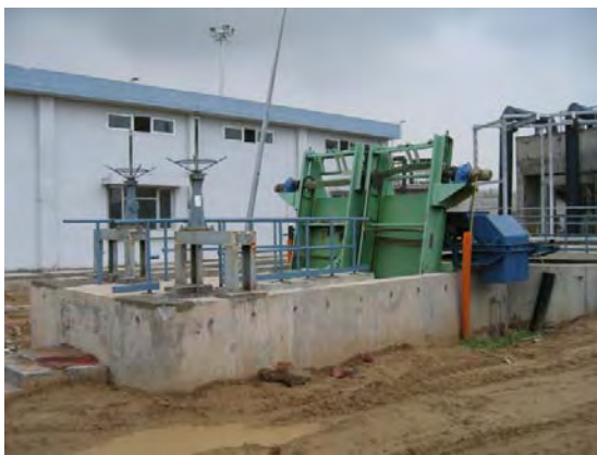
Coarse screen at intake
