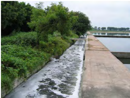
Effluent channel from polishing pond
