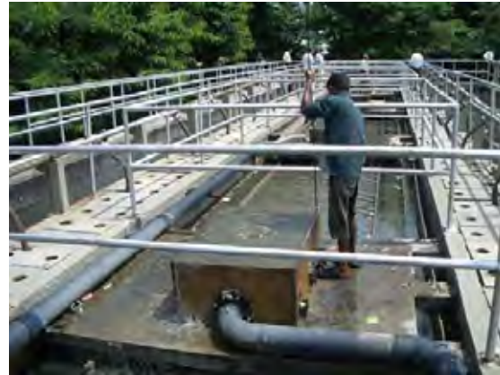
Cleaning of choked distribution at UASB
