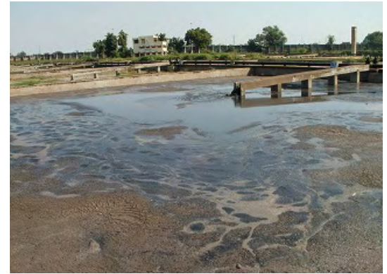
Sludge drying beds
