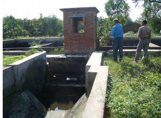
Mixing point of treated water and wastewater
