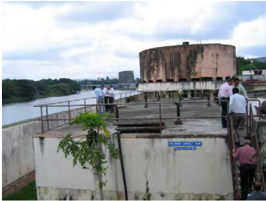
Chlorine contact tank
