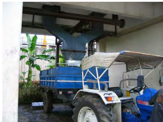
Dewatered sludge loaded in tractor trolley
