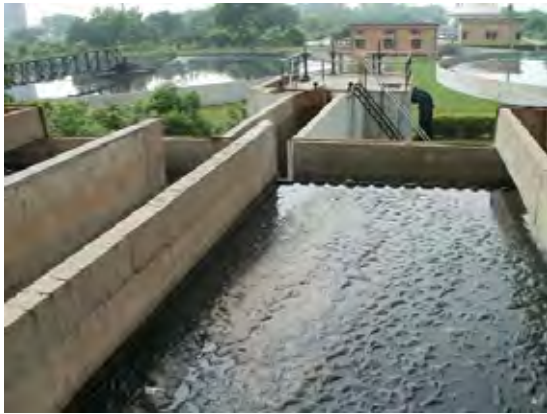
In Grit channel deposition of grit is observed
