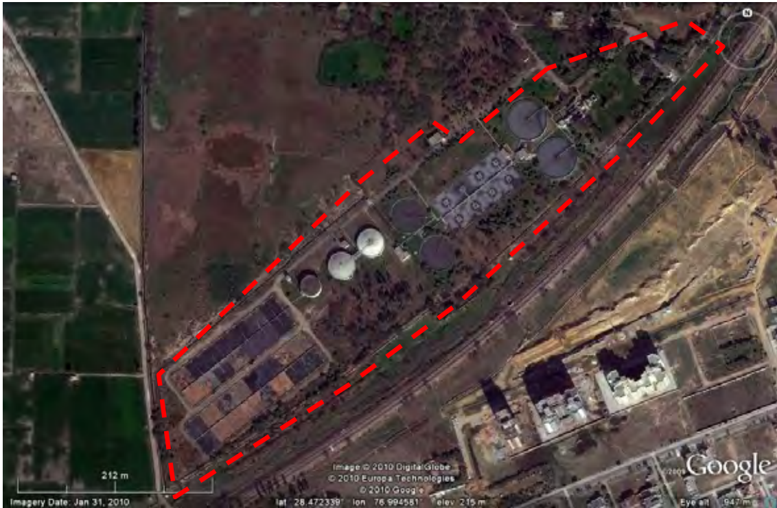
Figure 12 Location of Gurgaon 68MLD STP
