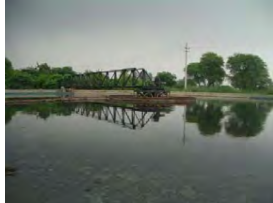
Primary settling tank
