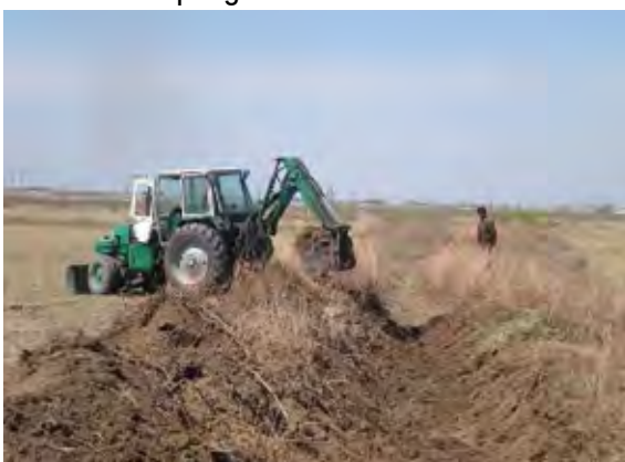
Canal maintenance by excavator of WUA
