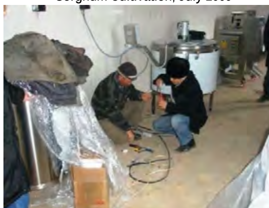
Installation of Milk Processing Equipments
