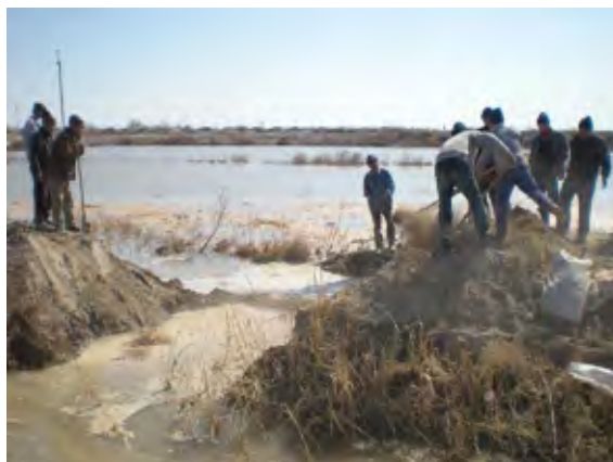
Canal maintenance by WUA, March 2009
