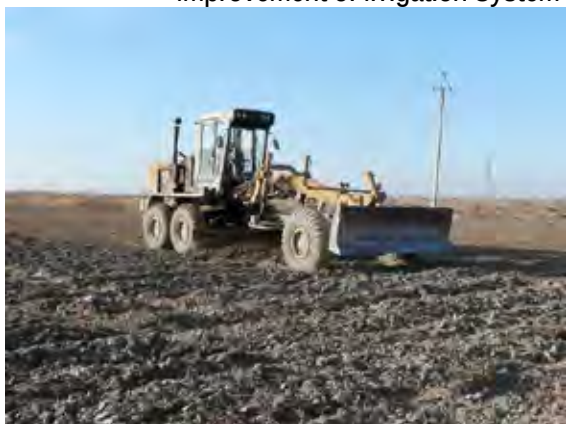
Land Leveling by Local Sub-contractor
