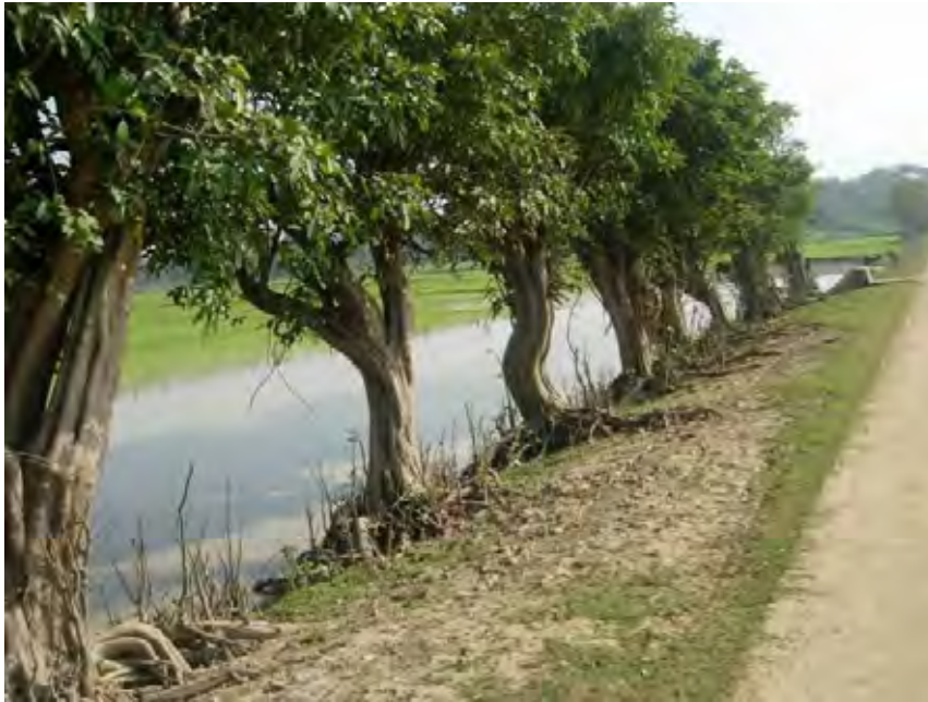
Figure 5.13: Trimming plantation of Karas plant beside a submersible embankment
