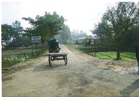
Hazipur Bazar Intersection
