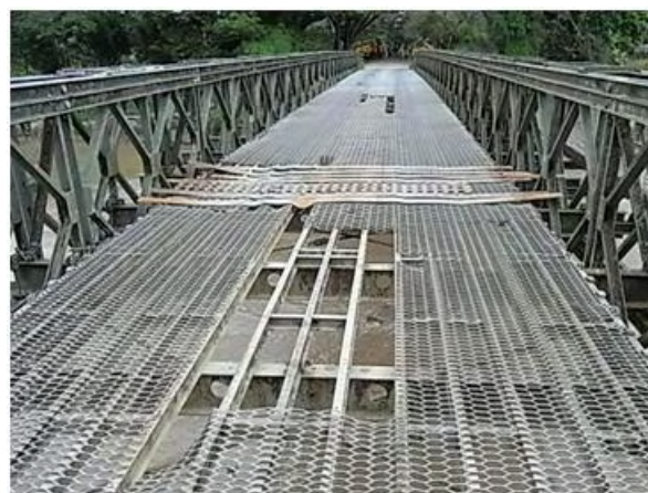
Photograph 1 Full View of the Angabanga Bridge Photograph 2 Damage to the Bridge Deck
