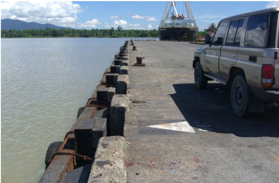
Photograph 6.4 The Current State of Berth 1
