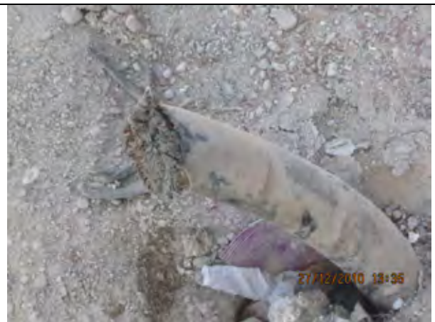
Cable Cut on the Street
