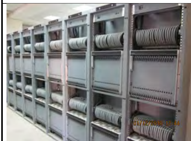
NGN Multi-Service Access Nodes (MSAN)
