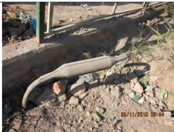
Cable Joint in the Street
