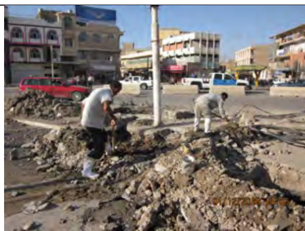
Telephone Cable Maintenance works on the Street
