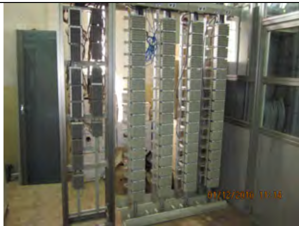
DWDM Digital Distribution Frame (DDF)
