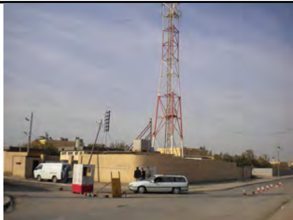
Switching Station Building
