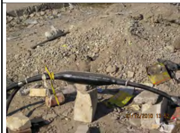
Cable Joint in the Street
