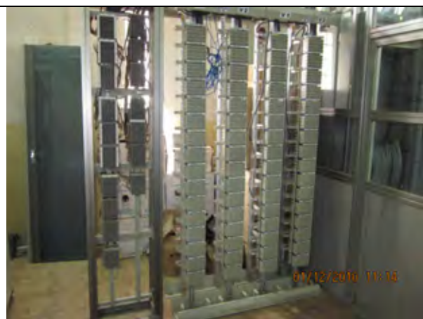
DWDM Digital Distribution Frame (DDF)
