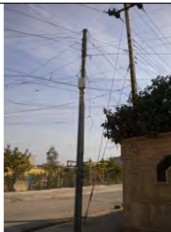
Telephone Pole with Distribution Box
