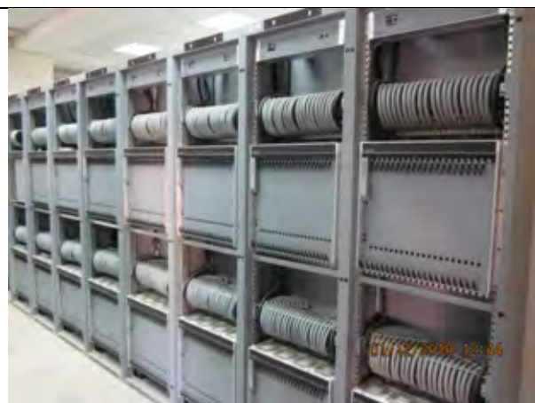
NGN Multi-Service Access Nodes (MSAN)
