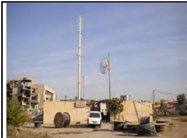
Switching Station Building
