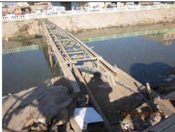
Cables Crossing a Small River over Small Bridge
