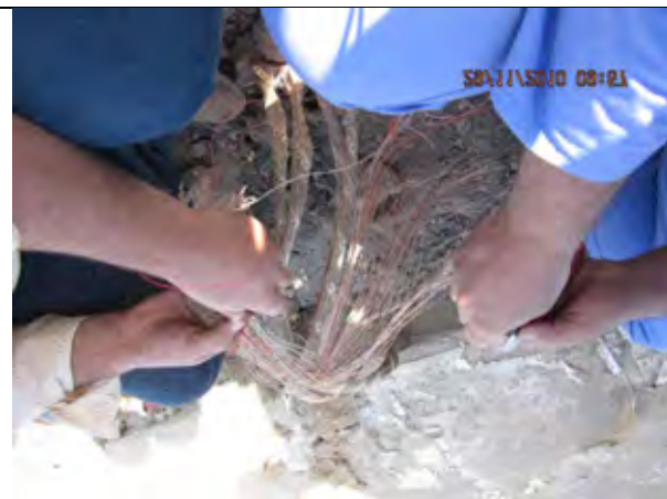
Cable Jointing Work
