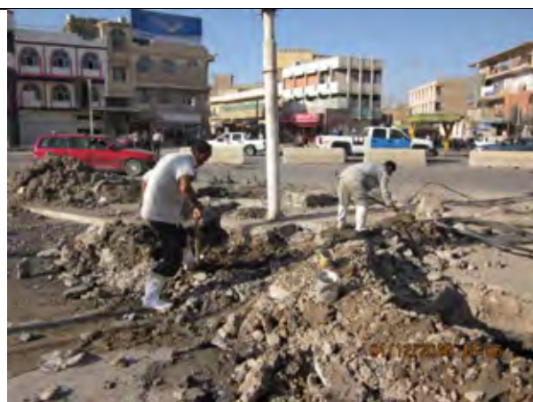
Telephone Cable Maintenance works on the Street
