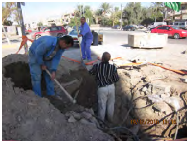
Cable Maintenance Work
