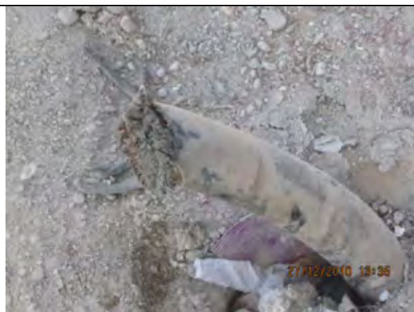
Cable Cut on the Street
