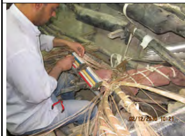
Cable Jointing Works inside Manhole
