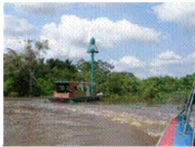
Planned Construction Site for New Coal Terminal
