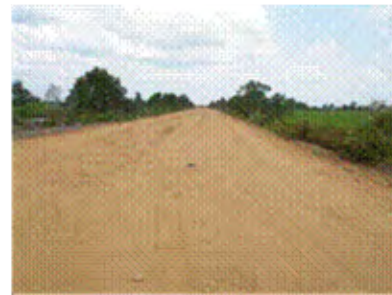
Access Road to New Coal terminal (under construction)
