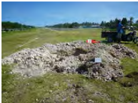
Full view of Test Pit
