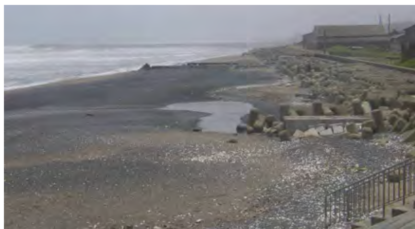
Photo 7.3 Two Months Later Work on Jinkouji Beach (5 June, 2008)
