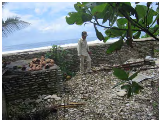
Photo 5.39 Cemented-Rock Seawall at Private Residence
