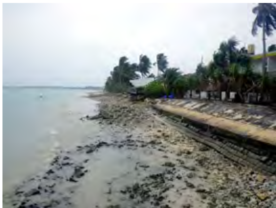
Photo 5.24 A Seawall Implemented as a Public Work - the Mixed Vertical/Sloping Seawall in front of Vaiaku Lagi Hotel
