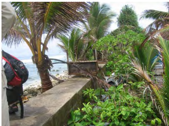
Photo 5.38 Concrete Seawall at Private Residence
