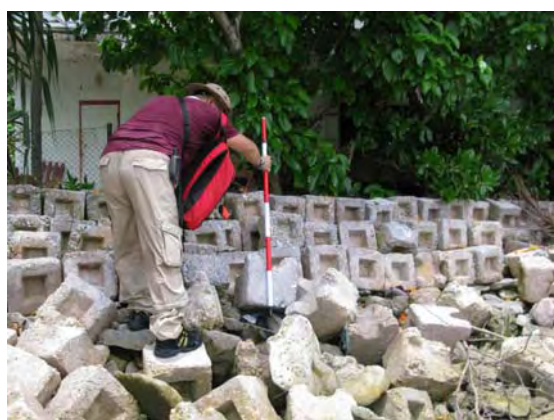
Photo 5.10 Close-up View of Catalina Ramp
