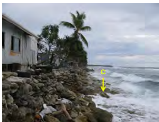
Photo 5.37 Private Seawall of Stacked-up Beachrock Fragments and Tyres
