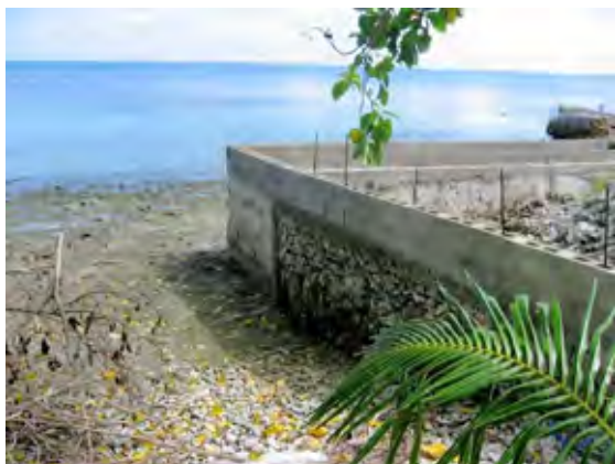
Photo 5.30 A Privately-Implemented Seawall – The Lower and Upper Parts Constructed with Gabions and Coping Concrete, Respectively
