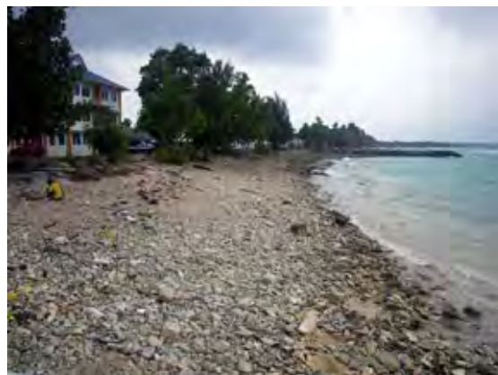
Photo 5.19 The Southern Side of Small Hotel Jetty
