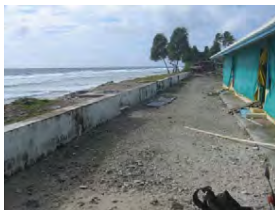
Photo 5.35 Concrete seawall in front of Church
