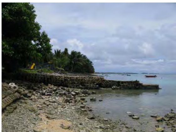
Photo 5.22 A Jetty Constructed with Recycled Concrete Blocks
