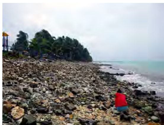
Photo 5.9 Seawall on the Southern Side of Catalina Ramp
