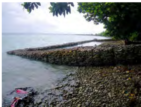
Photo 5.33 A Privately-Implemented Seawall – only Gabion Work Has Been Completed
