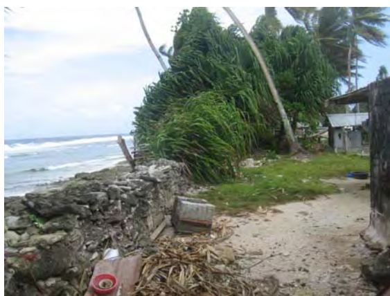
Photo 5.34 Private Seawall of Stacked-up Beachrock Fragments
