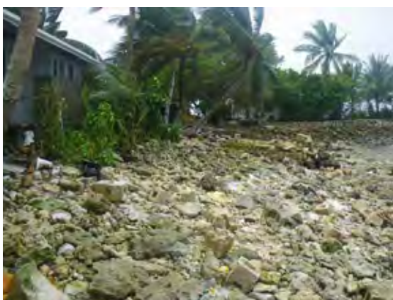
Photo 5.8 Seawall on the Northern Side of Catalina Ramp
