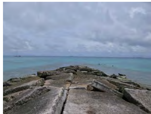
Photo 5.6 The Top of the Ramp
