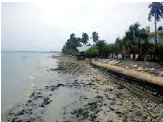
Photo 5.18 The Northern Side of Small Hotel Jetty
