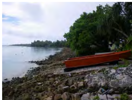
Photo 5.23 A Boat Landing Ramp
