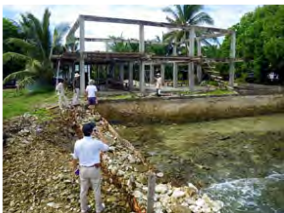
Photo 5.32 A Privately-Implemented Seawall – a Work Aimed at Land Development
