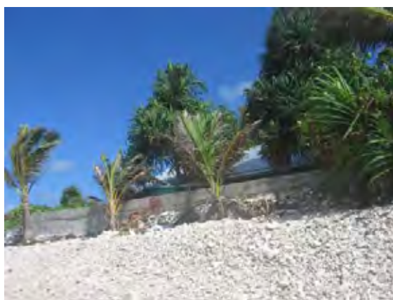
Photo 5.40 Concrete Seawall at Private Residence
