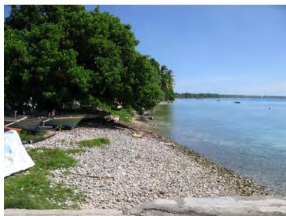
Photo 5.17 The Southern Side of Vaiaku Wharf
