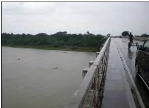
Photo 6.4.3 River Crossing Point (Madhumati River)
