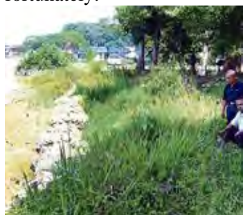
Emergency Work at Kg. Melayu
