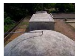
Digester, anaerobic baffled reactor (ARR) and anaerobic
