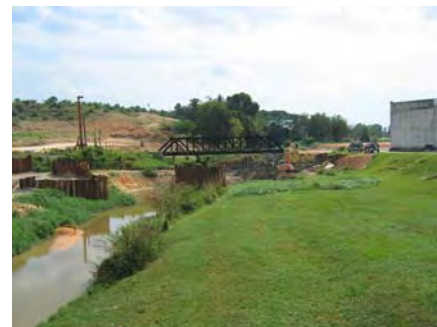
Railway Bridge on Gemas River
