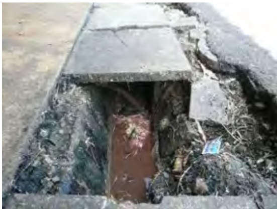
Wastewater from wet markets is one of the main sources of pollution load to the rivers. This picture was taken at the Labis wet market whereby wastewater together with some solid wastes from poultry slaughtering activities was discharged into a drain that flows into the Labis River right next to the market.
