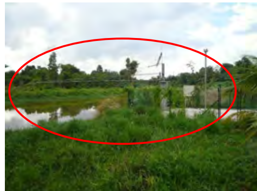
A flood warning siren was installed at Kpg. Raja Pagoh, adjacent to Pagoh Town, after the 2006/2007 flood.
