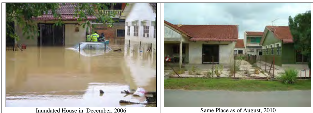
Figure 8.2.9 Inundated House and it Current Condition (Taman Sg. Gemas)
