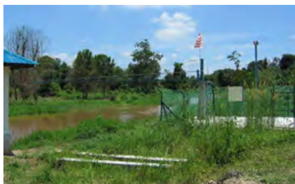
Flood Warning Siren at Pago, Muar
