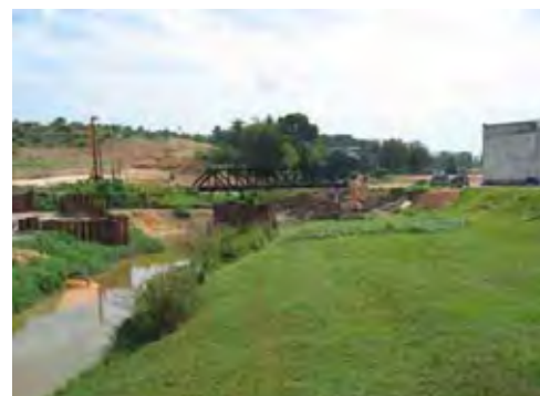
Railway Bridge on Gemas River
