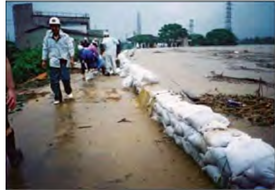
Sand bag Piling (Flood Fighting) 49
