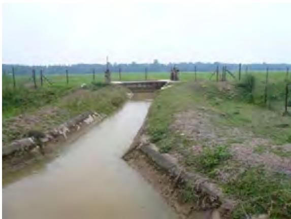
There are a number of irrigation schemes in the Pahang River Basin. This is the Paya Kertau Irrigation Scheme at Maran District.
