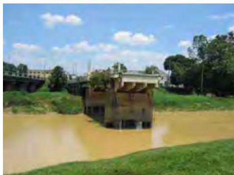
Abandoned old bridge on the Muar River at Kg. Kuning Patah
