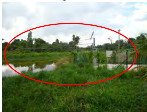
A flood warning siren was installed at Kpg. Raja Pagoh, adjacent to Pagoh Town, after the 2006/2007 flood.
