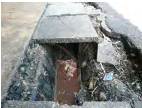
Wastewater from wet markets is one of the main sources of pollution load to the rivers. This picture was taken at the Labis wet market whereby wastewater together with some solid wastes from poultry slaughtering activities was discharged into a drain that flows into the Labis River right next to the market.
