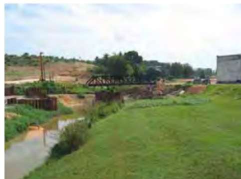
Railway Bridge on Gemas River
